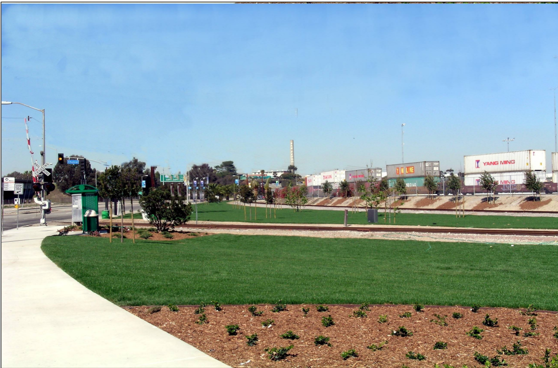
Same Picture with Above Ground Utilities Removed
