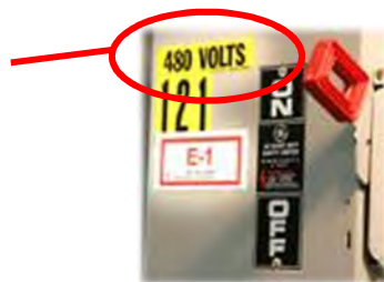
Voltage ID on OEM label
