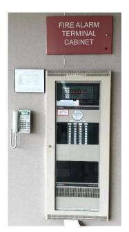
activated position, another alarm will be initiated, or in some cases, the panel will refuse to reset until all the alarms have been reset/cleared. A system reset is often required to clear supervisory conditions. A system reset does not usually clear trouble conditions; most trouble conditions will clear automatically when conditions are returned to normal.
