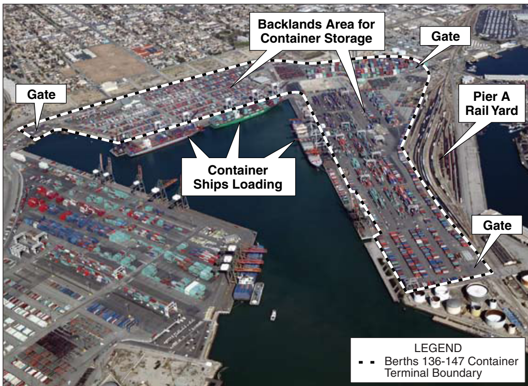
Figure 1-2. Existing Container Terminal
