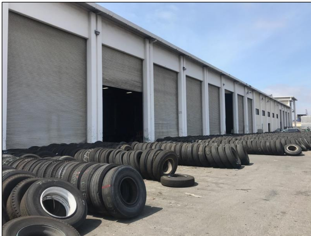
Figure 14. North façade of the Container Equipment Maintenance Building/Office Tower, view southwest (SWCA, 2018).
