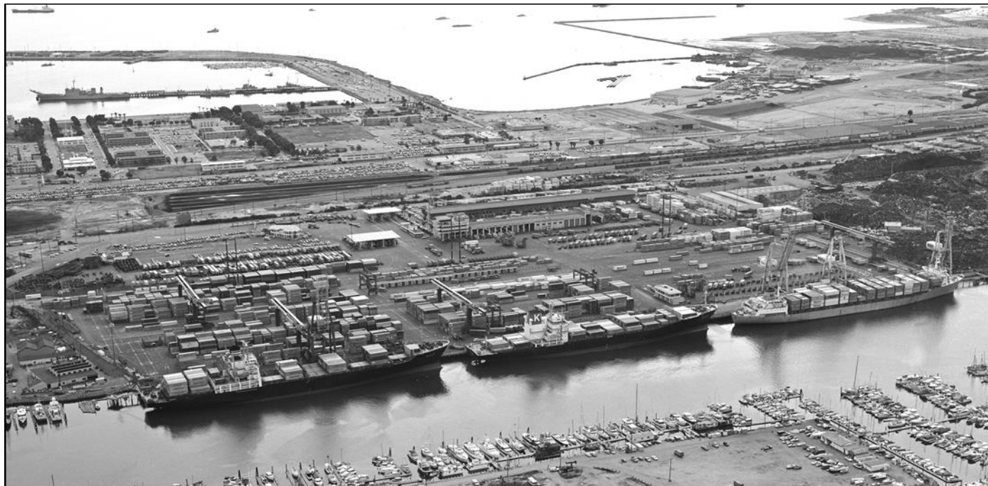
Figure 4. Historical aerial image of the Matson Container Terminal, view southwest, 1982 (Source: Port of Los Angeles).
