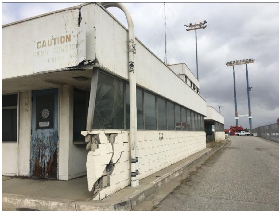
Figure 10. East façade of the Gate Office Building, view north (SWCA, 2018).
