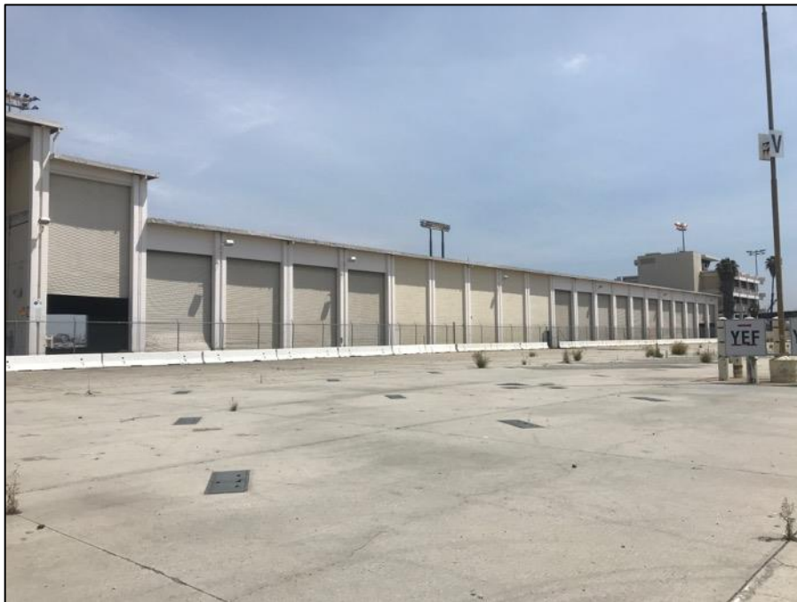
Figure 12. South façade of the Container Equipment Maintenance Building/Office Tower, view northeast (SWCA, 2018).
