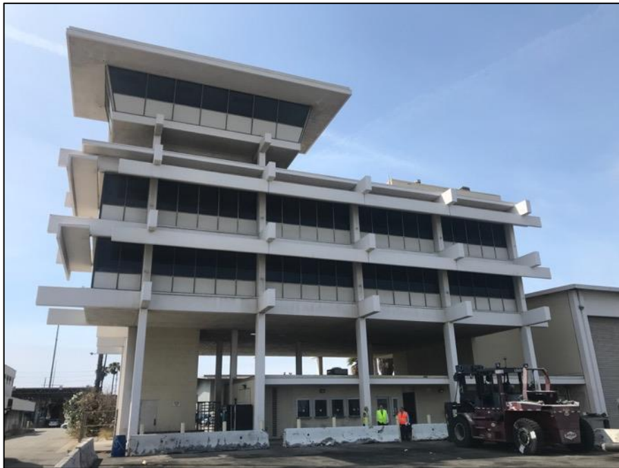
Figure 19. North façade of the Office Tower, view south (SWCA, 2018).
