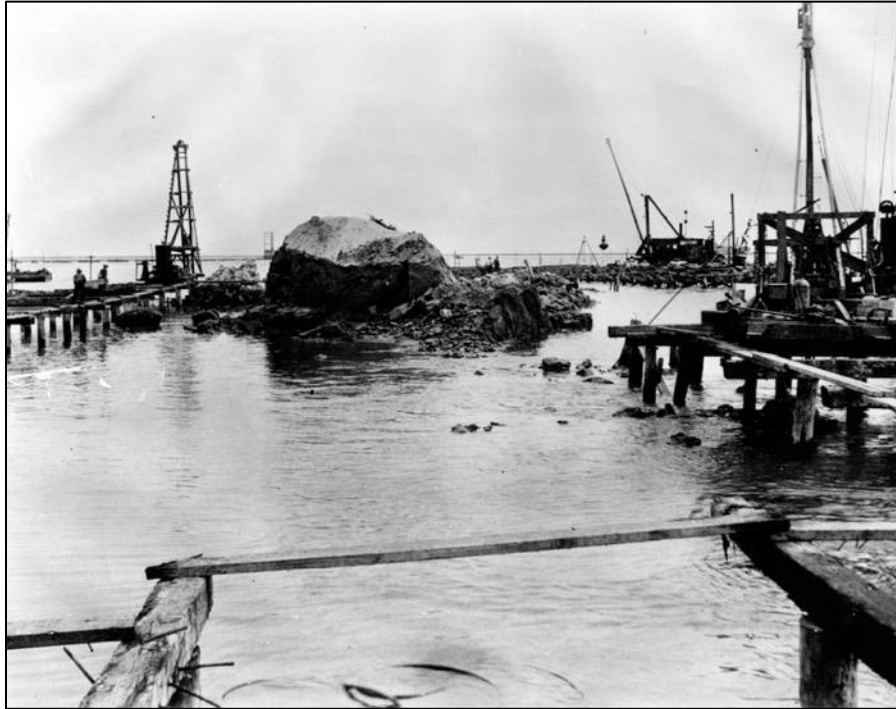
Figure 28. Demolition of Dead Man's Island, dredging and infilling to create Terminal Island ca. 1920 (Los Angeles Water and Power Associates Photo Archive).
