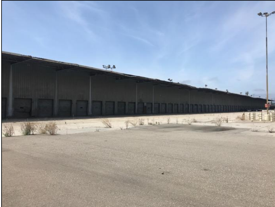
Figure 24. North façade of the Consolidated Freight Station, view southeast (SWCA, 2018).
