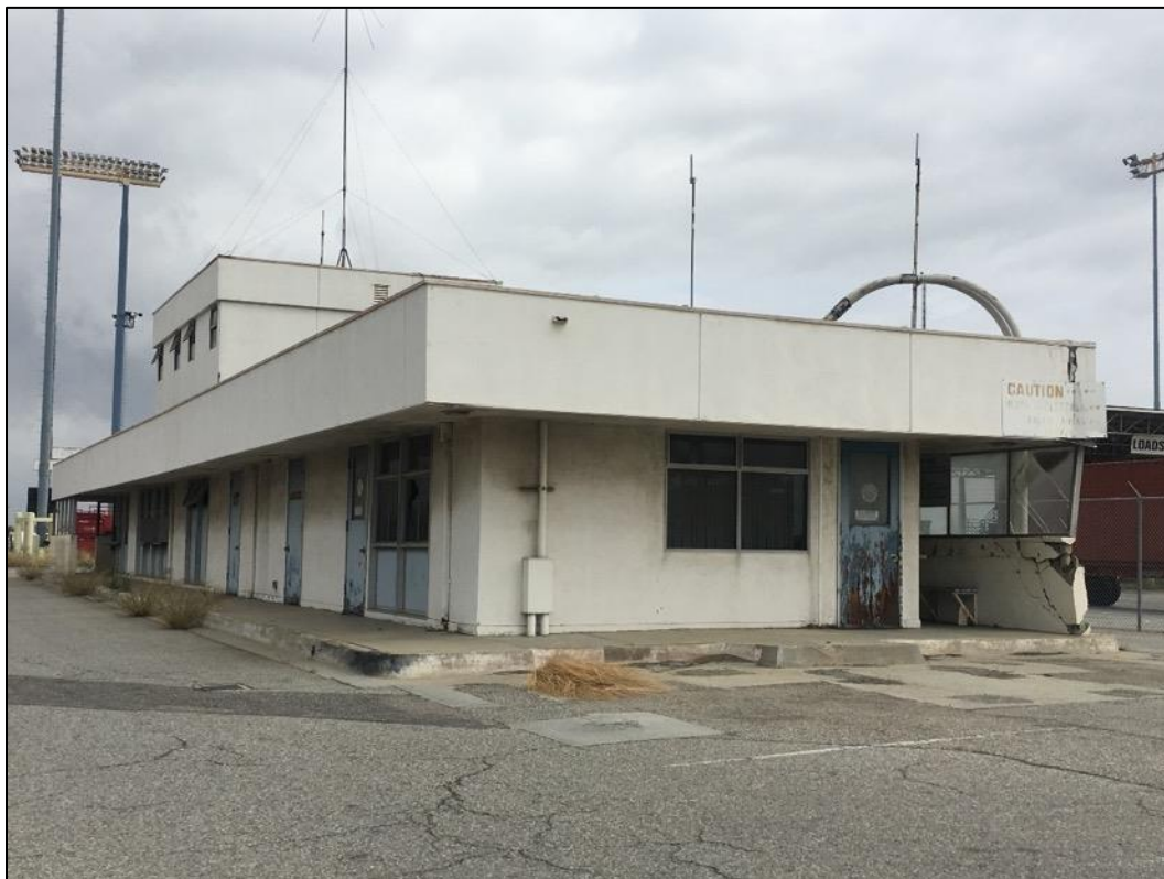
Figure 4. West (left) and south (right) façades of the Gate Office Building, view north (SWCA, 2018).
