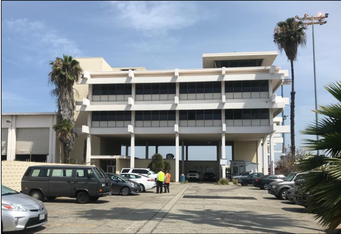
Figure 16. Primary (south) façade of the Office Tower, view north (SWCA, 2018).
