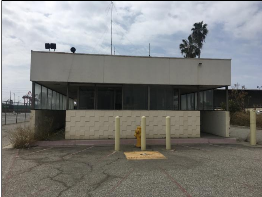
Figure 9. North façade of the Gate Office Building, view south (SWCA, 2018).
