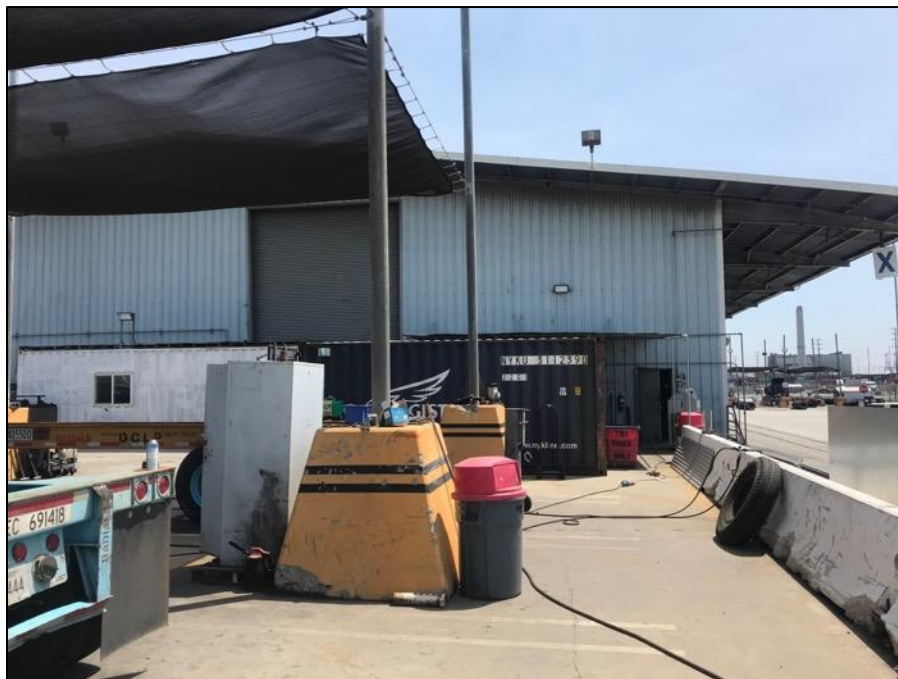
Figure 23. West façade of the Consolidated Freight Station, view east (SWCA, 2018).
