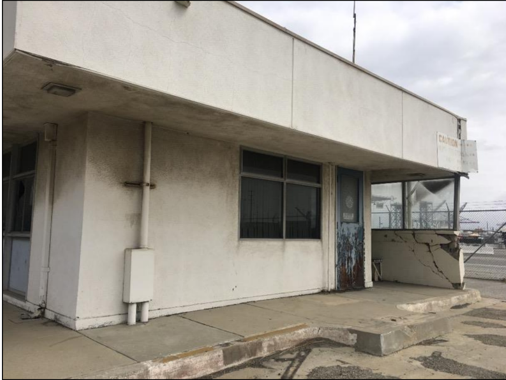
Figure 5. South façade of the Gate Office Building, view northeast (SWCA, 2018).
