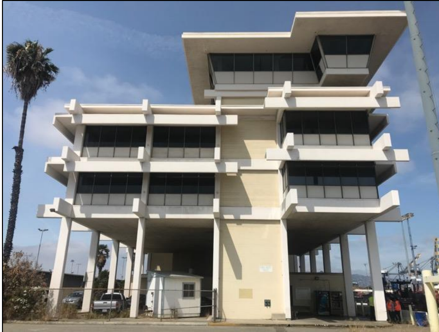
Figure 20. East façade of the Office Tower, view west (SWCA, 2018).
