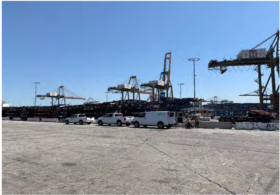
Photograph 3: Geophysical survey set up at Boring B14. View looking northeast.
