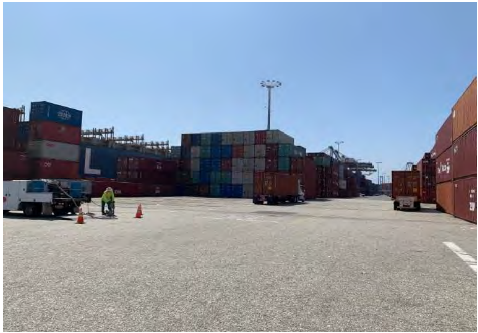
Photograph 5: Coring pavement at Boring B12 prior to drilling. View looking southeast.
