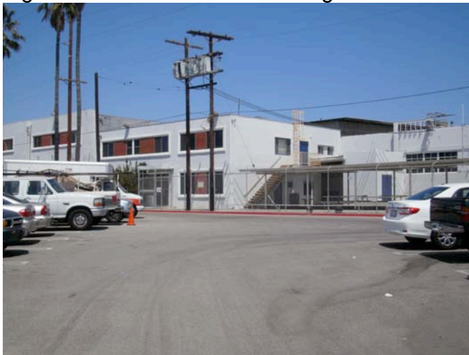
Figure 4. Starkist Historic Building
