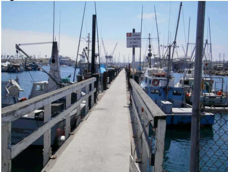
Figure 1. Berth 167 in Fish Harbor.
