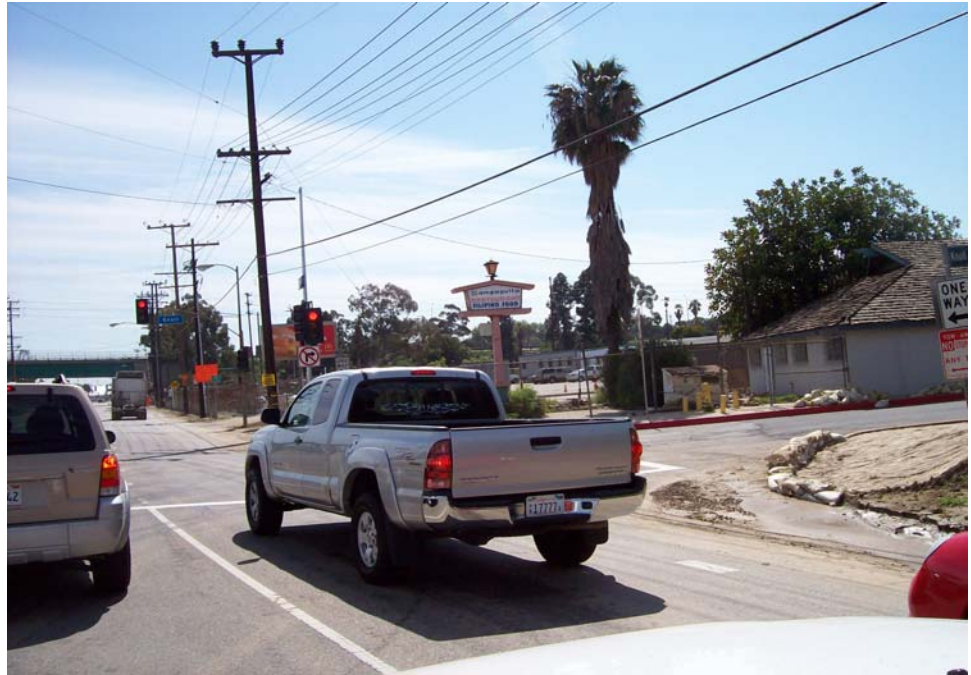
Photograph No. 17: Looking south along North Front Street, within Area C.
