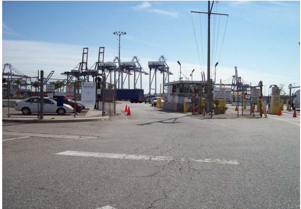
Photograph No. 13: Looking south at TraPac, within Area C.
