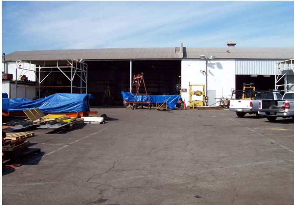
Photograph No. 3: Looking west along Marine Avenue (at 211 Marine Avenue), within Area A.
