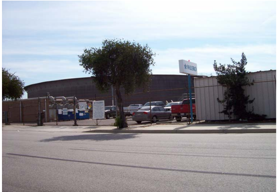
Photograph No. 9: Looking southeast from A Street at Valero, within Area B.
