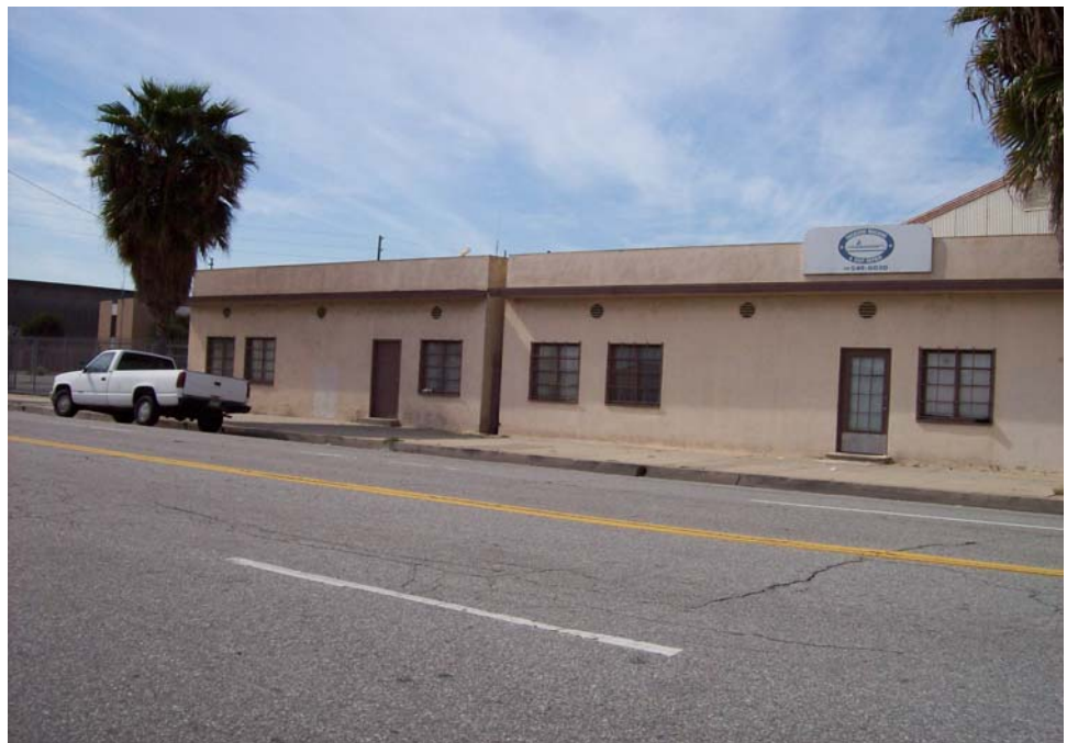
Photograph No. 8: Looking southwest from Avalon Boulevard at the Dockside Machine and Ship Repair facility, within Area B.
