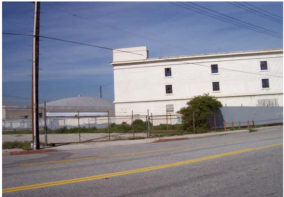
Photograph No. 4: Looking northwest along North Fries Avenue, within Area A.
