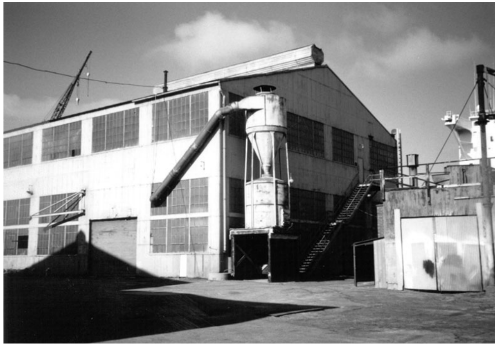
Photograph 2. Sawdust silo at north elevation
