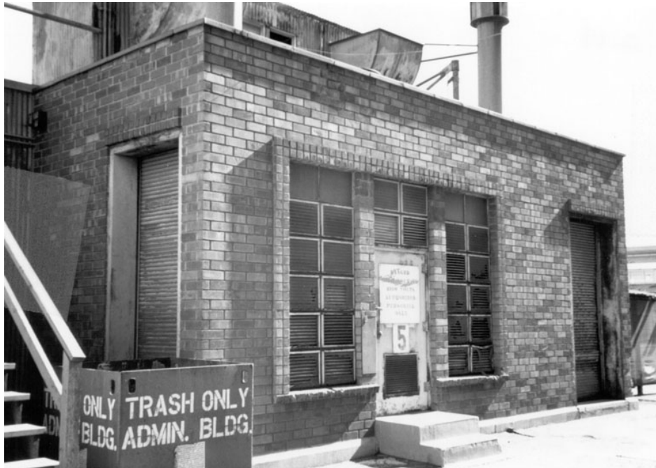
Photograph 2. Substation, southwest elevation
