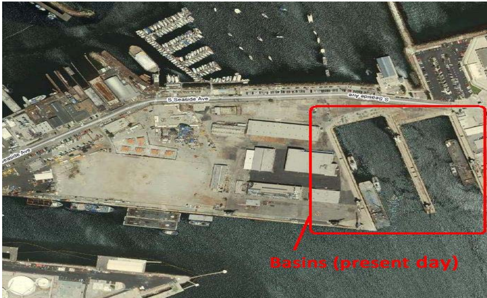
Figure 5 –This present-day photo (2009) shows the basins and complete removal of the floating dry docks.
