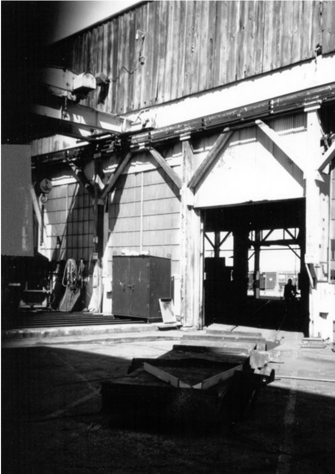
Photograph 3. Cart on track running through building
