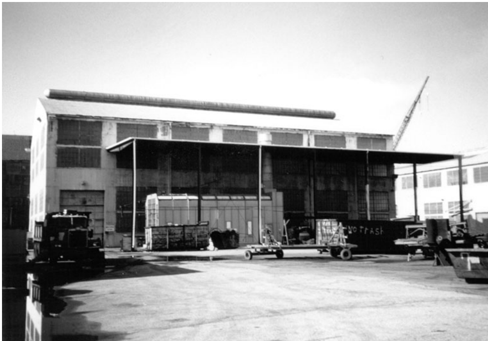
Photograph 2. Metal shelter at rear of building
