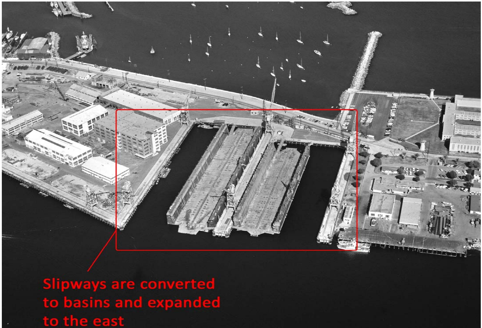
Figure 4 - This 1964 photo illustrates the 1959–1961 expansion of the basins to east, the complete removal of the shipbuilding slipways, and construction of steel and concrete piers.
