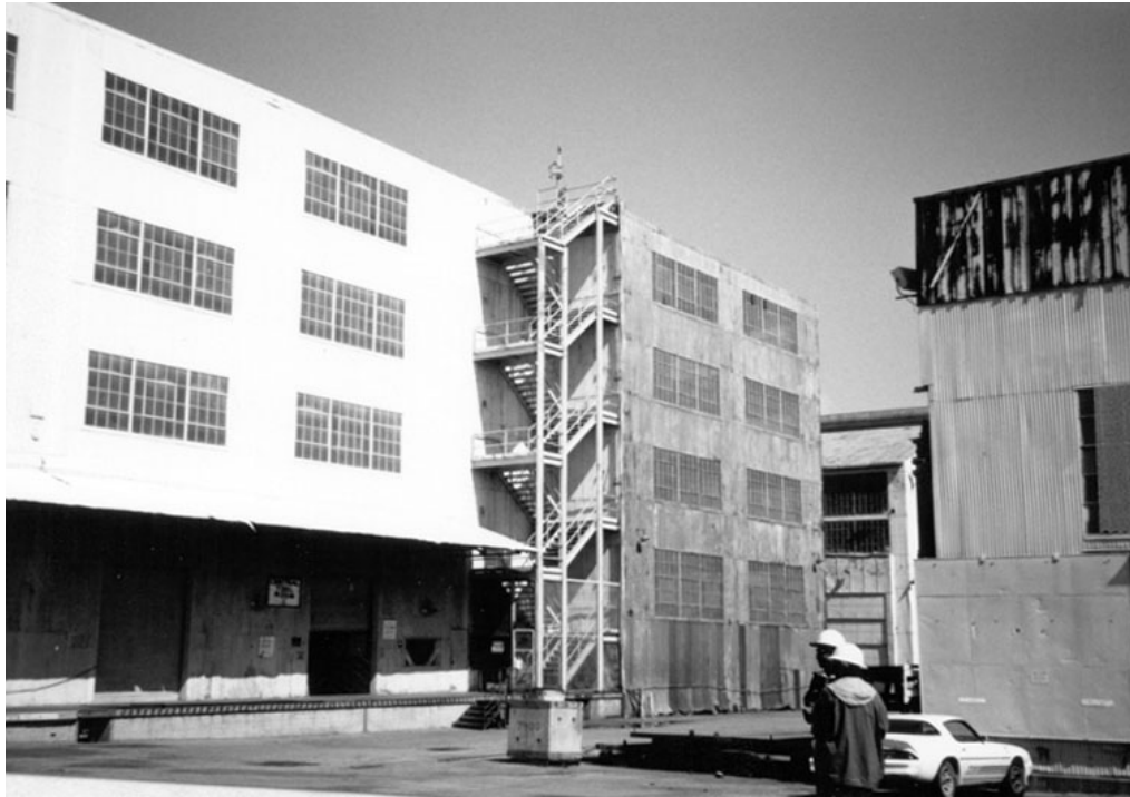
Photograph 2. Exterior metal stairs
