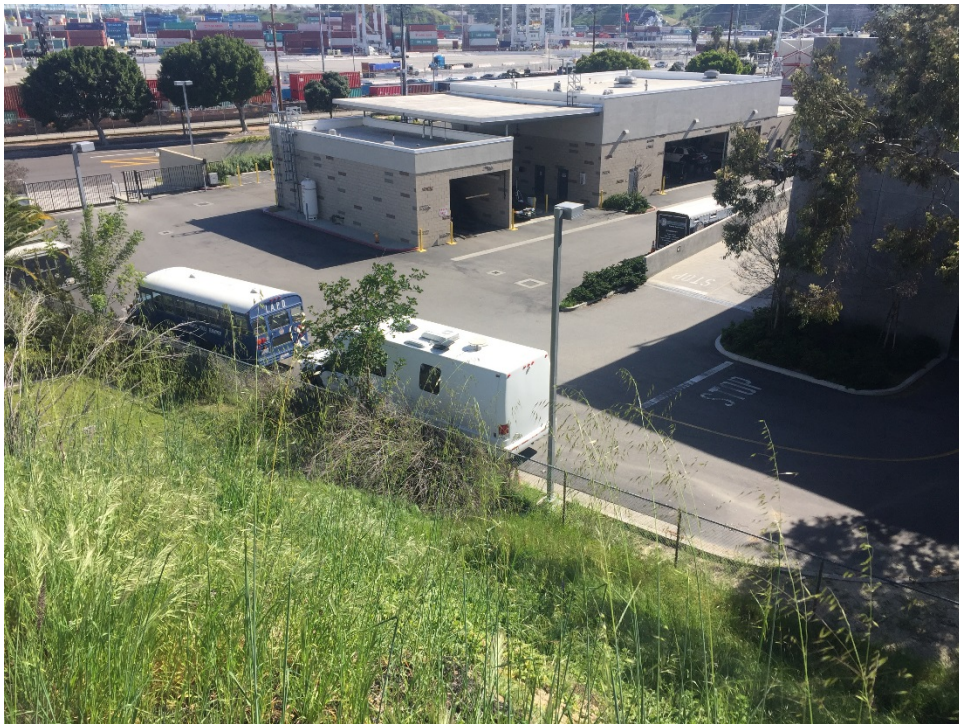
Photo 14 – The police station to the south of the southwestern end of the Property.
