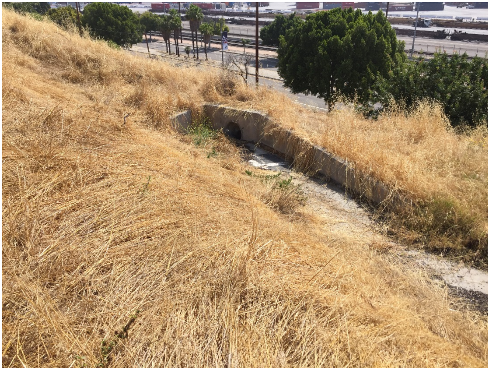
Photo 28 – Stormwater drain on the Property.
