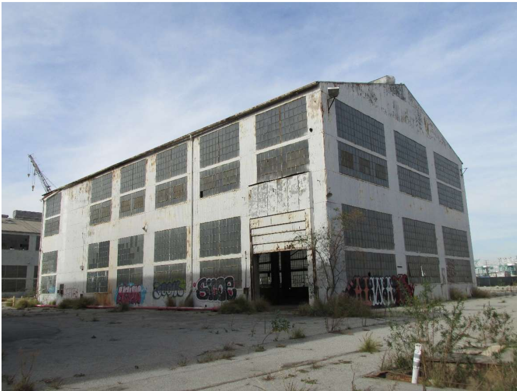
Figure 11. Shop #9, Southeast Elevation, IMG_9432
