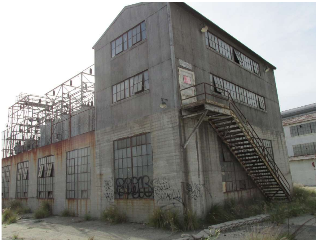
Figure 5. Transportation Shop #4, Northeast Elevation, IMG_9465
