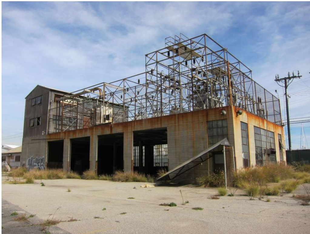
Figure 4. Transportation Shop #4, Southwest Elevation, IMG_7863
