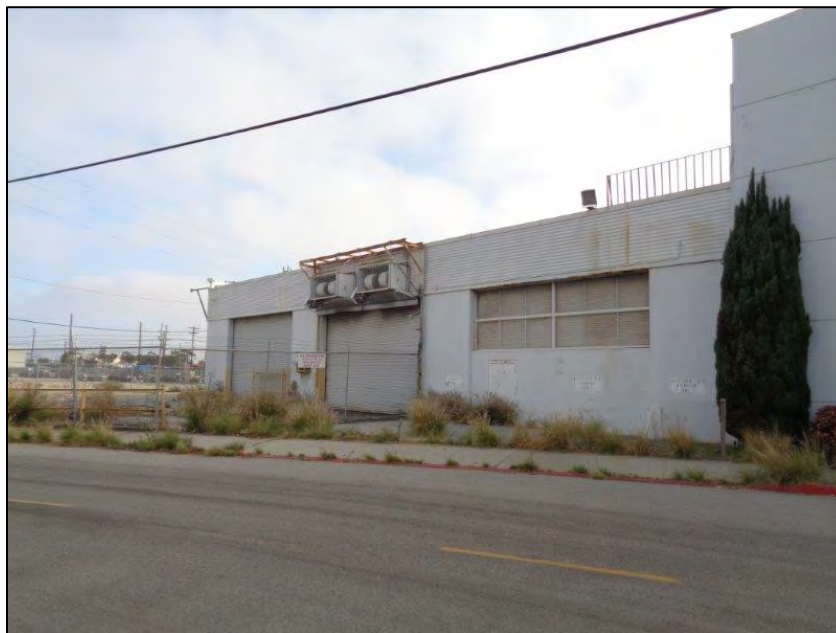
Figure 5-8. Star-Kist Plant No. 4, primary (west) elevation, detail of northern volume, camera facing northeast.
