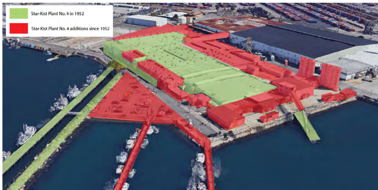
Figure 7-7. Birds-eye view of Star-Kist Plant No. 4 in 2018, with green overlay denoting extant portions of the 1952 building and red noting additions since 1952, camera facing northeast.
