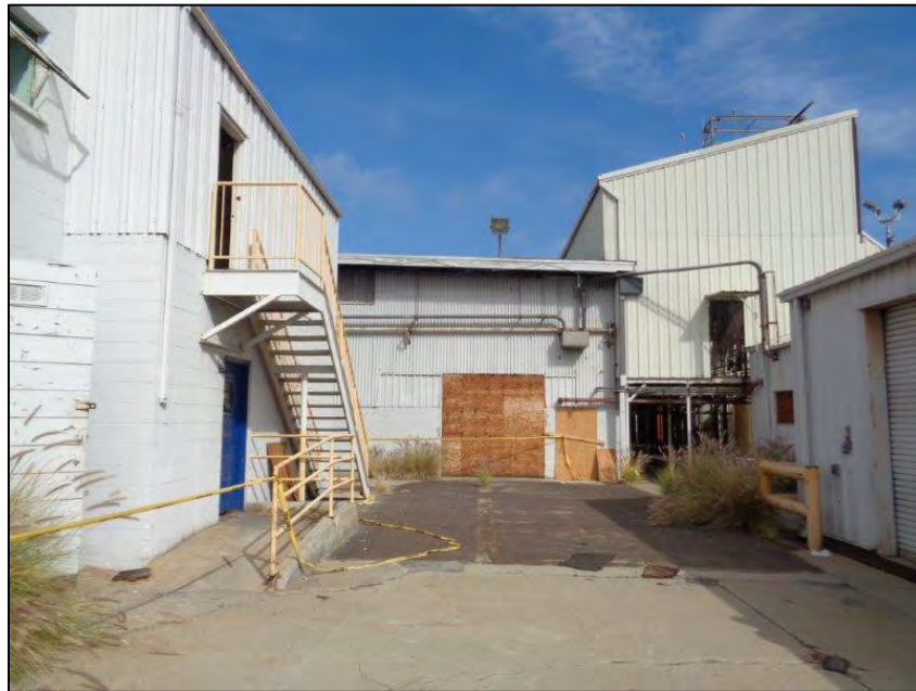
Figure 5-24. Star-Kist Plant No. 4, rear (east) elevation, detail of ancillary two buildings/structures (left, with staircase; right, with roll-up door) and warehouse/manufacturing building (center), camera facing north.
