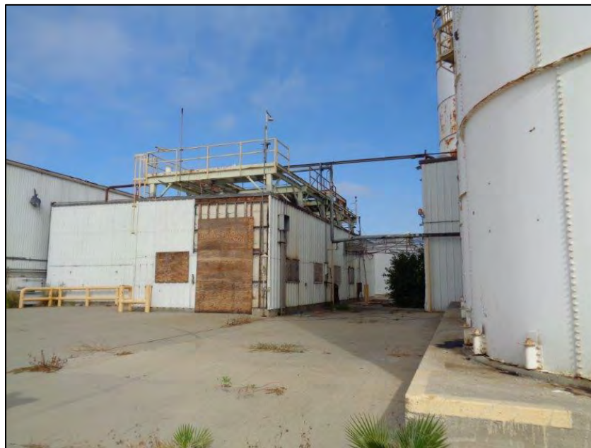
Figure 18: Star-Kist Plant No. 4, south and rear (east) elevations, southeast corner of Plant No. 4, camera facing north. ICF, 2018.
