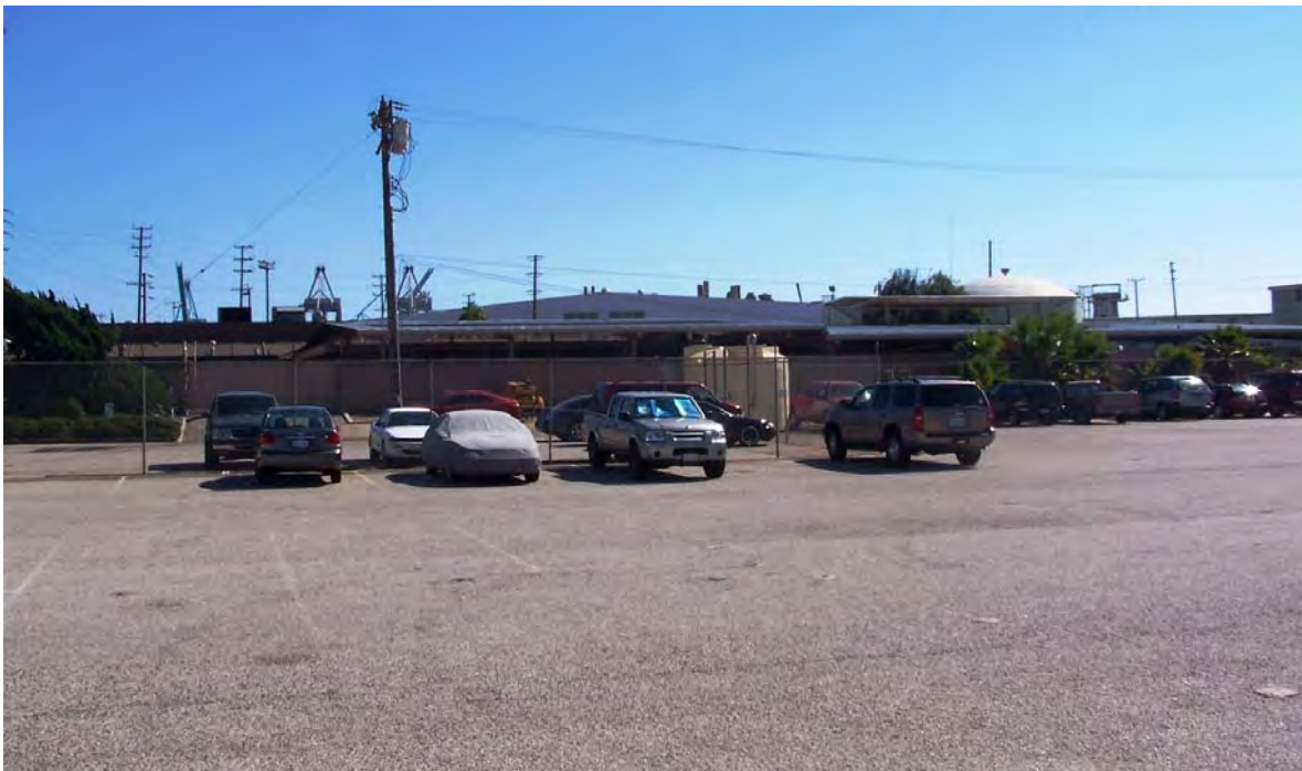
Photo 25. Looking south at the northern elevation of the Animal Care Facility
