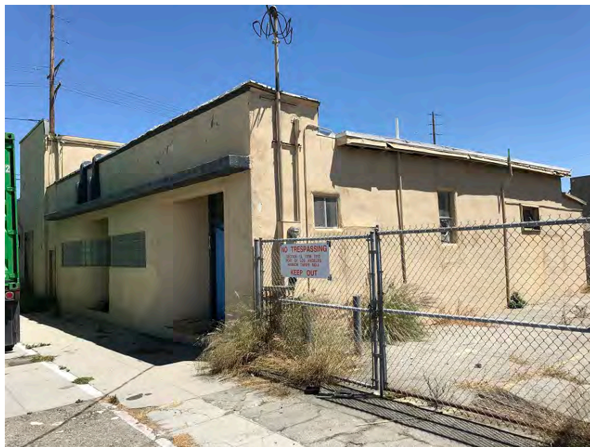
Figure 10-3. Nakamura Multi-Use Building, primary (west) elevation and south elevation, camera facing northwest.
