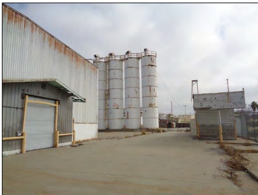
Figure 5-18. Star-Kist Plant No. 4, south elevation, southeast corner including tanks, camera facing east. ICF, 2018.
