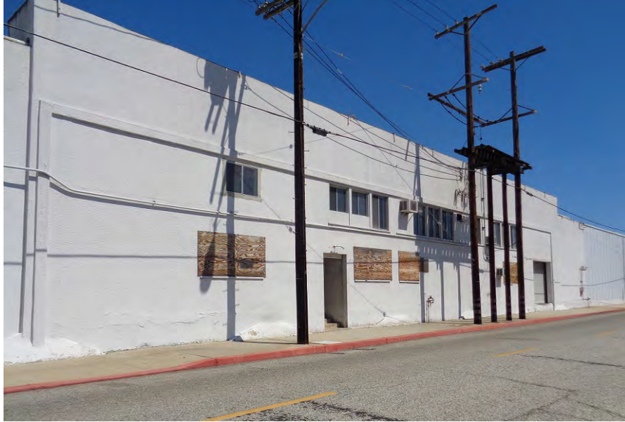
Figure 10-8. Cannery Block, west elevation showing an older building with Moderne elements, camera facing south.
