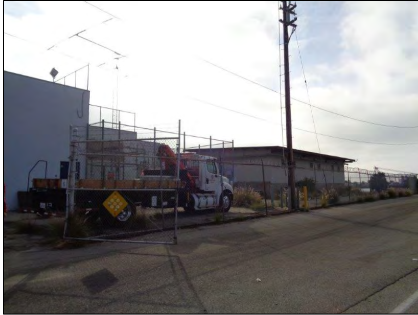
Figure 5-14. Star-Kist Plant No. 4, primary (west) elevation, detail of southwest corner of Plant, showing gated electrical area and detached building, camera facing southeast.
