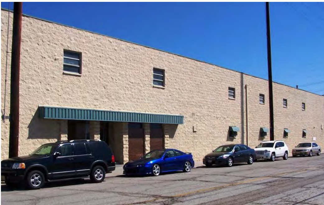
Photo 28. Looking southeast across Tuna Street at the western elevation of the Pilot Plant
