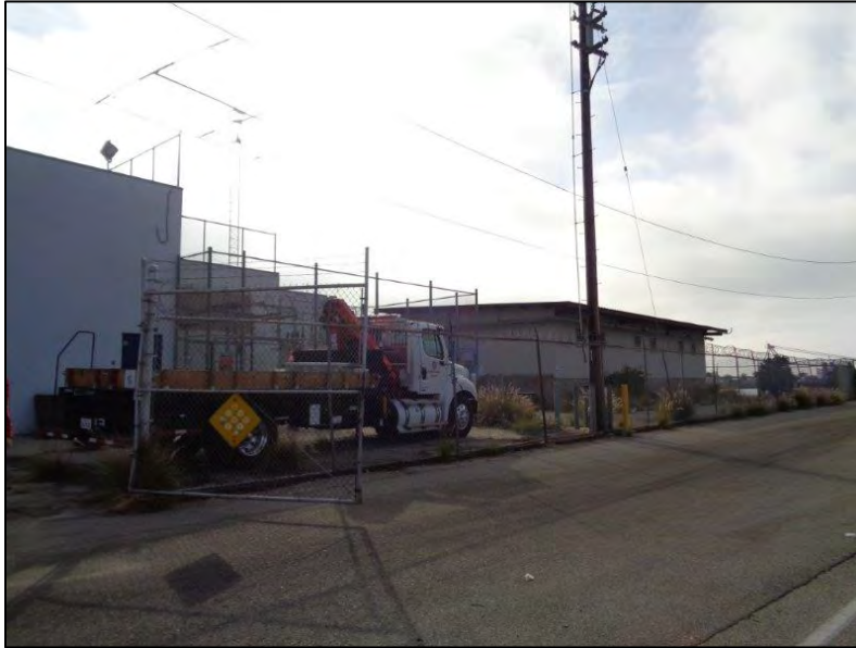
Figure 13: Star-Kist Plant No. 4, primary (west) elevation, detail of southwest corner of Plant No. 4, showing gated electrical area and detached volume, camera facing southeast. ICF, 2018.
