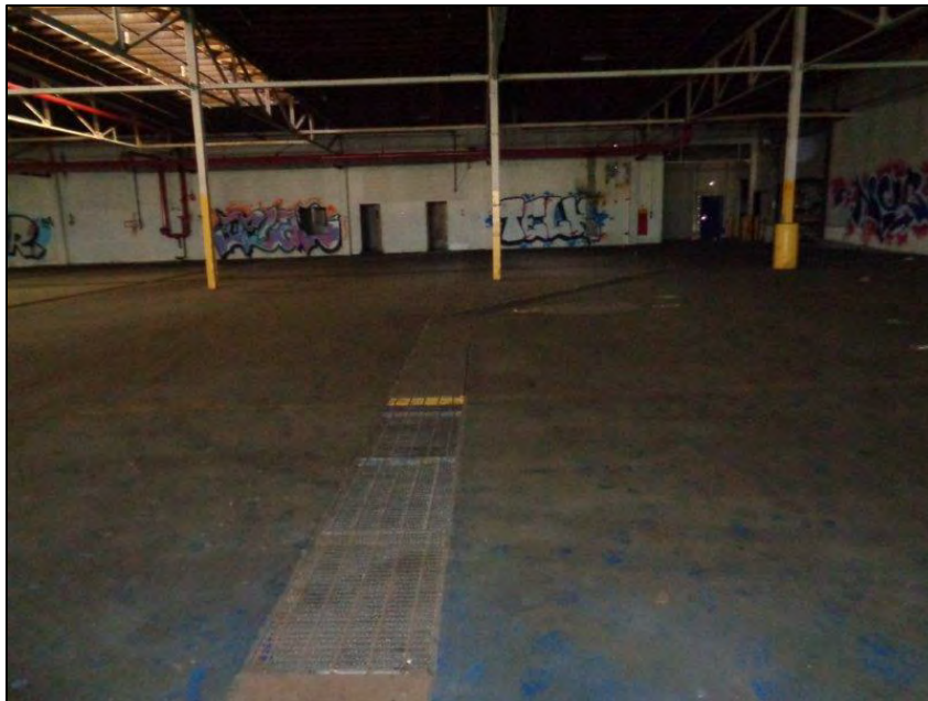
Figure 5-29. Star-Kist Plant No. 4, interior, warehouse/manufacturing area showing drains in floor, camera facing east.
