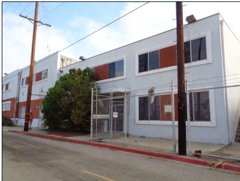
Figure 10: Star-Kist Plant No. 4, primary (west) elevation, detail of fifth volume from the north, camera facing northeast. ICF, 2018.
