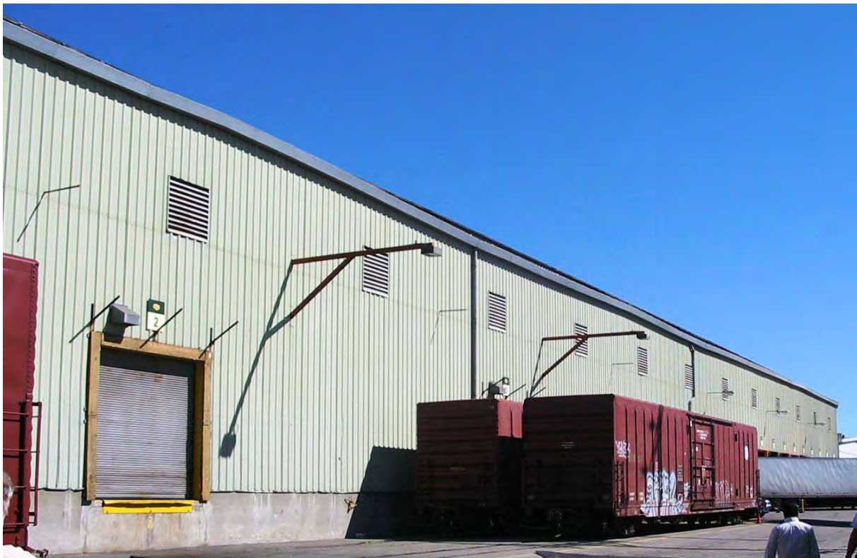
Photo 22. Looking southeast at the western elevation of the Warehouse/Distribution Center
