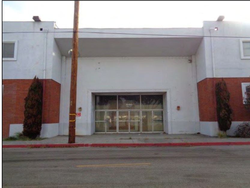
Figure 3: Star-Kist Plant No. 4, primary (west) elevation, detail of third volume from the north, entrance pylon, camera facing east. ICF, 2018.
