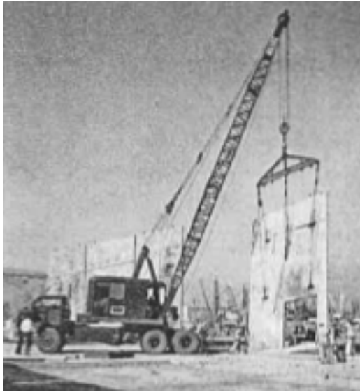
Figure 7-1. Construction of Star-Kist Plant No. 4.
