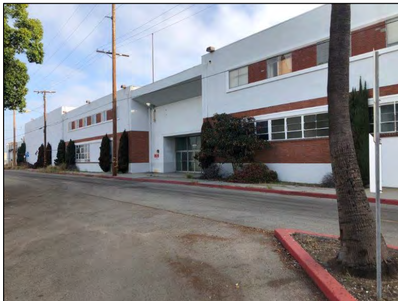
Figure 2: Star-Kist Plant No. 4, primary (west) elevation showing entrance, camera facing northeast. ICF, 2018.
