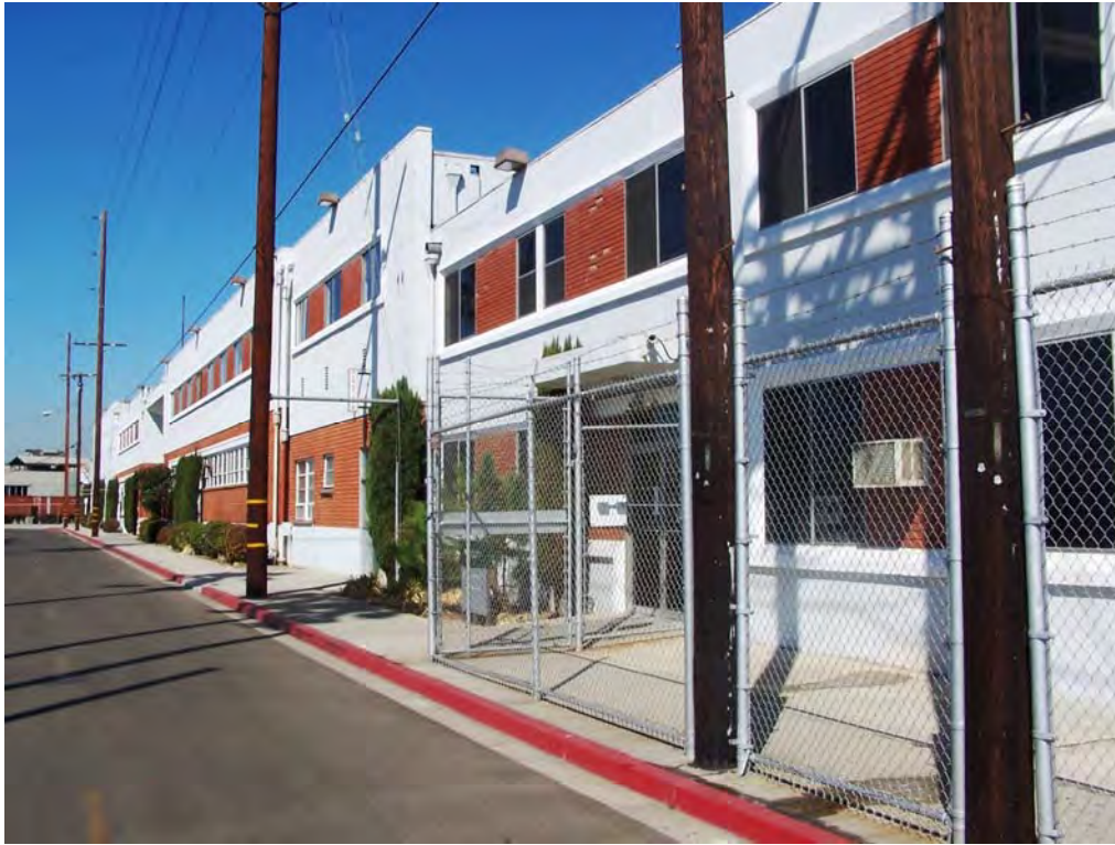
Photo 20. Looking northeast at the center of the western elevation of original plant
