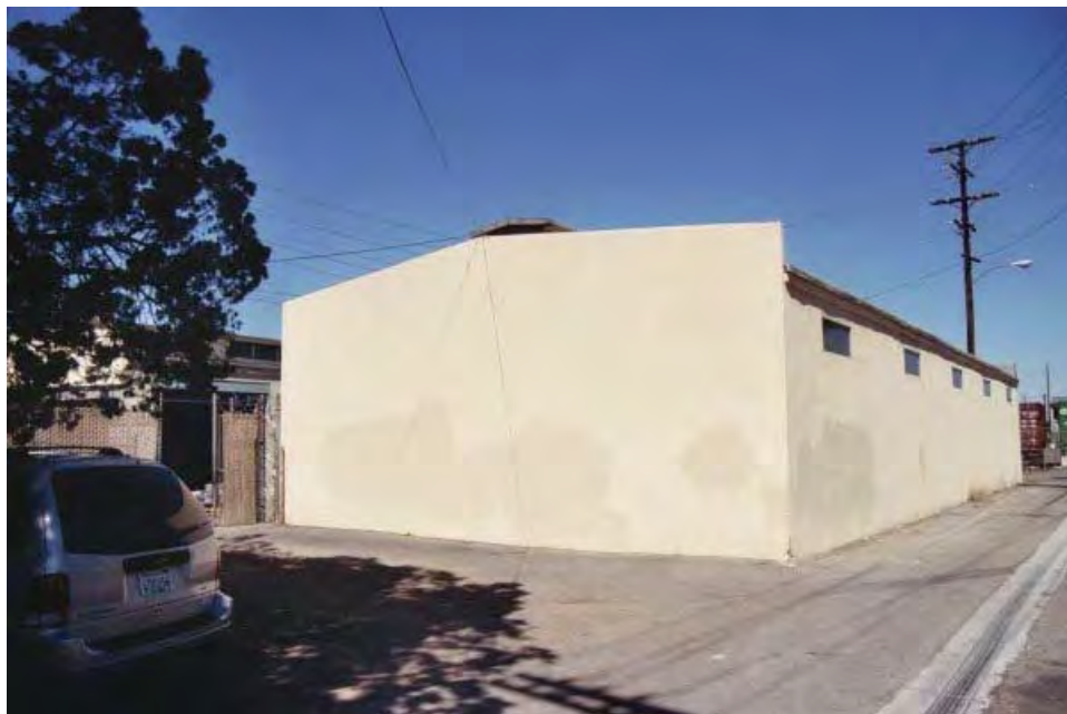
Photo 29. Looking northeast at the western elevation of the Net Repair Sheds (“Boneyard”)
