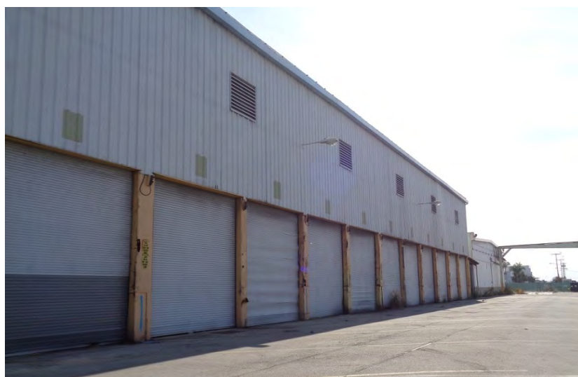
Figure 5-38. West elevation, Warehouse portion of facility in foreground (left) and Cold Storage portion in the distance (right), camera facing south.
