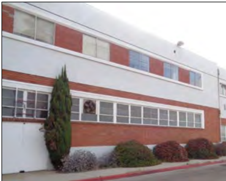
Figure 6: Star-Kist Plant No. 4, primary (west) elevation, detail of third building from the north, south wing, camera facing east. ICF, 2018.
