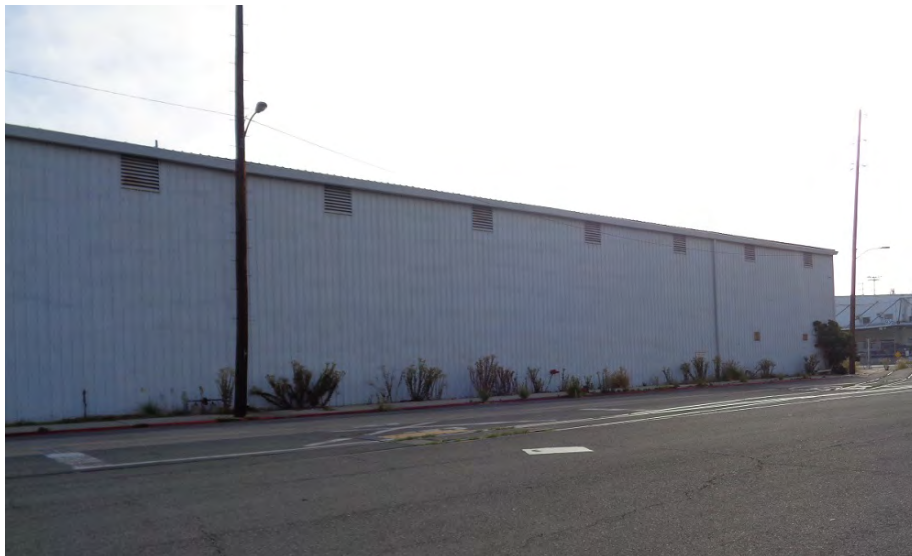
Figure 5-34. West elevation, camera facing southwest.
