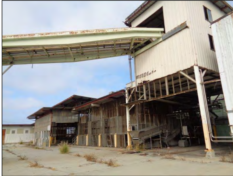
Figure 15: Star-Kist Plant No. 4, south elevation, southwest corner of Plant, showing tuna import bridge, camera facing northwest. ICF, 2018.
