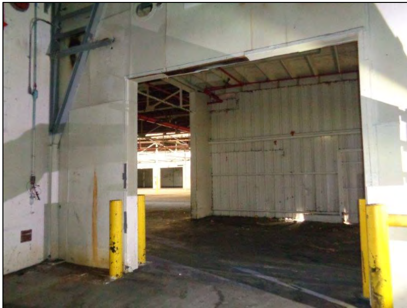
Figure 5-31. Star-Kist Plant No. 4, interior, warehouse/manufacturing area, camera facing east. ICF, 2018.
