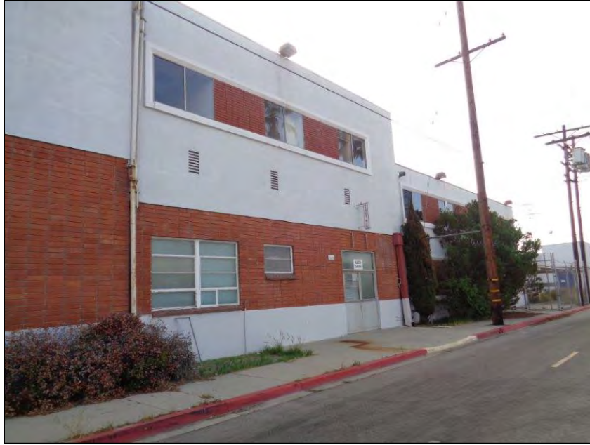
Figure 5-10. Star-Kist Plant No. 4, primary (west) elevation, detail of fourth volume from the north, camera facing southeast.
