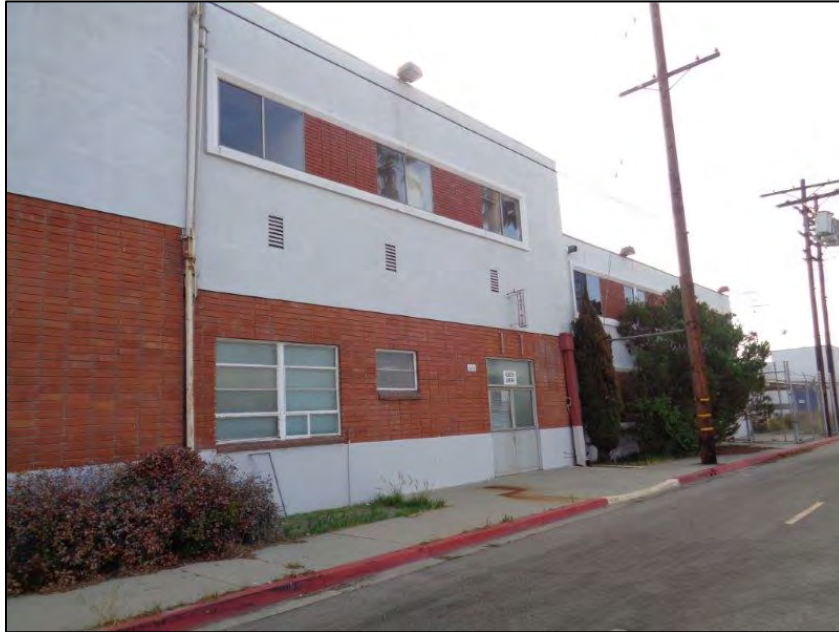
Figure 9: Star-Kist Plant No. 4, primary (west) elevation, detail of fourth volume from the north, camera facing southeast. ICF, 2018.
