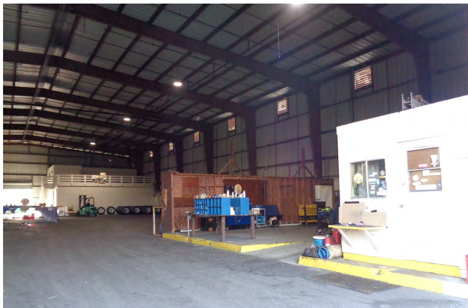
Figure 5-35. Interior, camera facing south.
