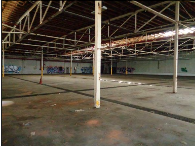
Figure 27: Star-Kist Plant No. 4, interior, warehouse/manufacturing area showing drains in floor, camera facing southeast. ICF, 2018.
