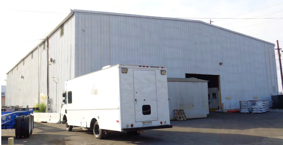
Figure 5-33. North and west elevations, camera facing south.
