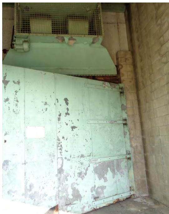
Figure 5-41. South elevation, Cold Storage portion of the facility, detail showing a cold storage door, camera facing northeast.
