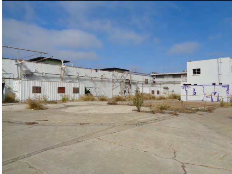
Figure 5-23. Star-Kist Plant No. 4, rear (east) elevation, southeast corner of Plant, detail showing rear of warehouse/manufacturing building (left) and ancillary building/structure (right [with purple graffiti]), camera facing northwest.
