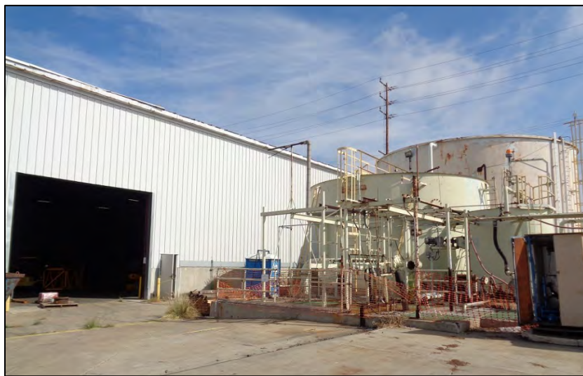
Photograph 4: South elevation, Cold Storage portion of the facility, camera facing northeast. ICF, 2018.
