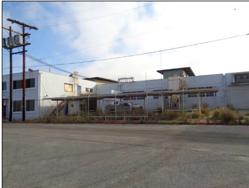
Figure 11: Star-Kist Plant No. 4, primary elevation, detail of lunch patio and recessed warehouse/manufacturing building, sixth volume from the north, camera facing northeast. ICF, 2018.
