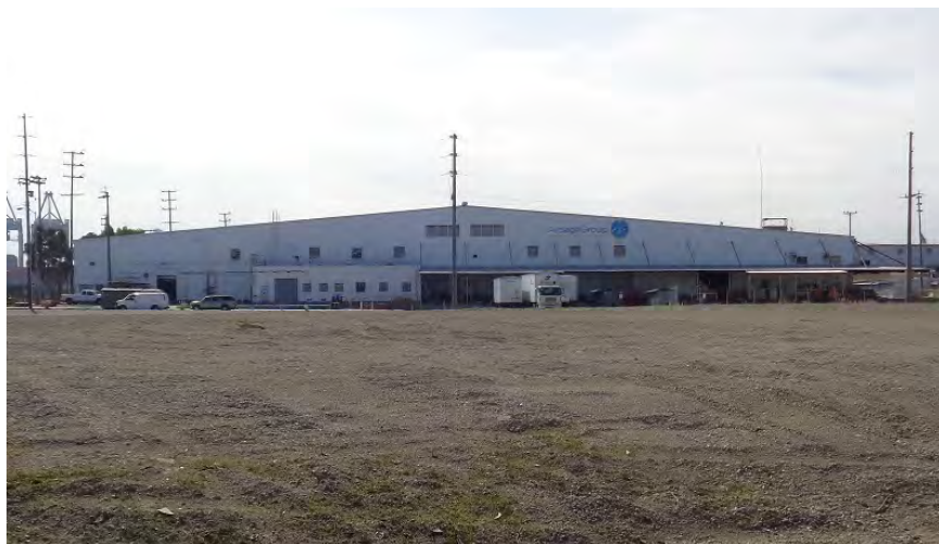
Figure 5-36. North elevation, Can Manufacturing Plant portion of facility, camera facing south.
