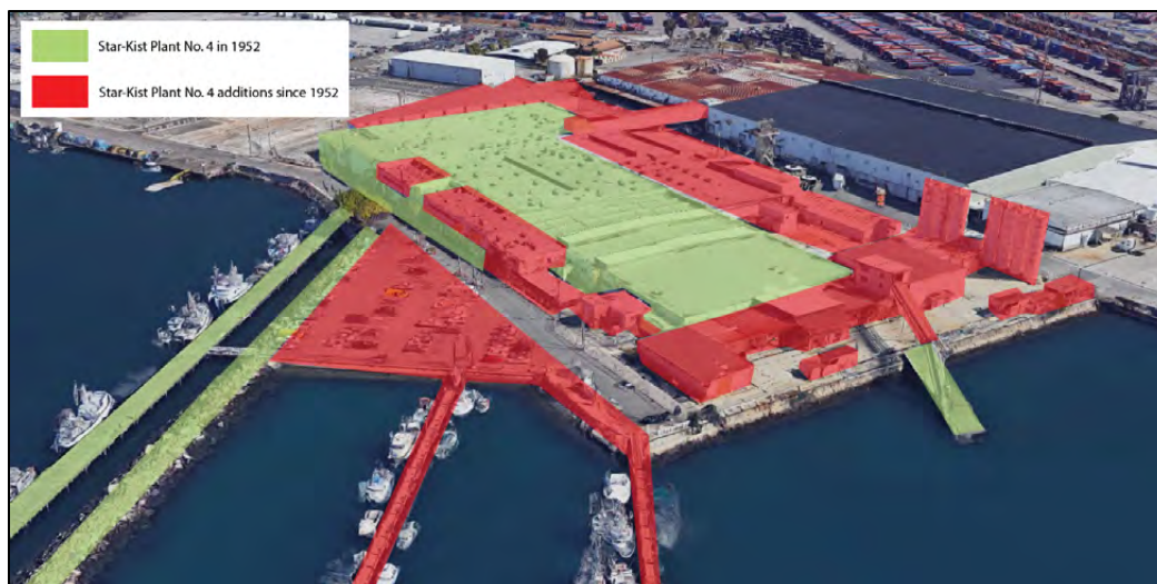
Figure 2-1. Birds-eye view of Star-Kist Plant No. 4 in 2018, with green overlay denoting extant portions of the 1952 building and red noting additions since 1952, camera facing northeast.
