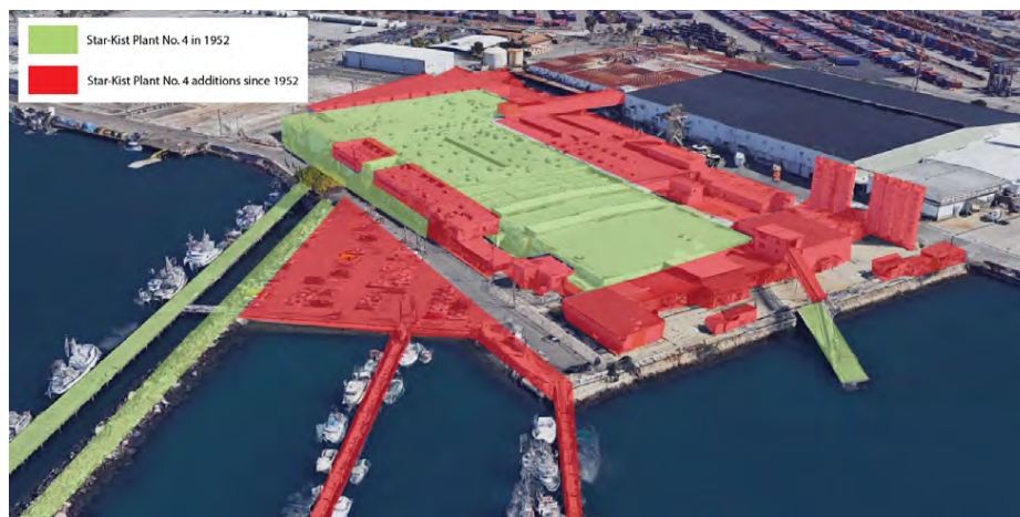
Figure 8-2. Birds-eye view of Star-Kist Plant No. 4 in 2018, with green overlay denoting extant portions of the 1952 building and red noting additions since 1952, camera facing northeast.
