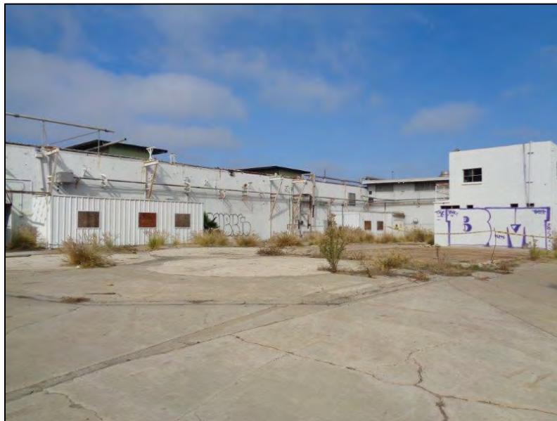
Figure 22: Star-Kist Plant No. 4, rear (east) elevation, southeast corner of Plant, detail showing rear of warehouse/manufacturing building (left) and ancillary building/structure (right [with purple graffiti]), camera facing northwest. ICF, 2018.
