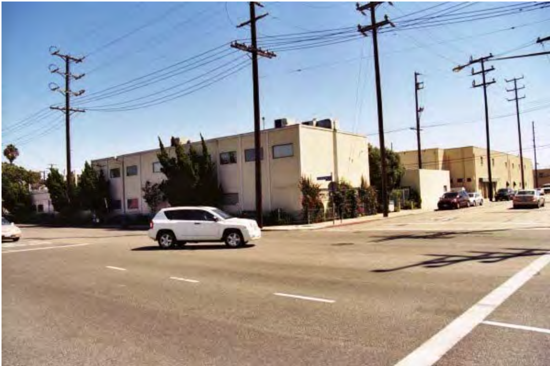
Photo 26. Looking southeast across Terminal Way at the northwestern corner of the Research Laboratory Complex
