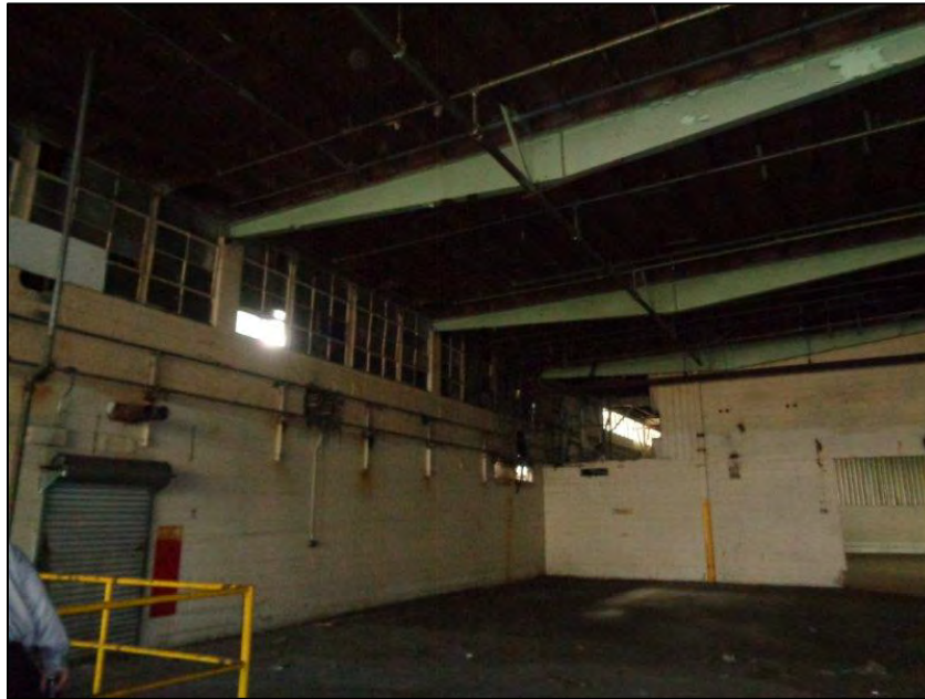
Figure 31: Star-Kist Plant No. 4, interior, warehouse. ICF, 2018.
