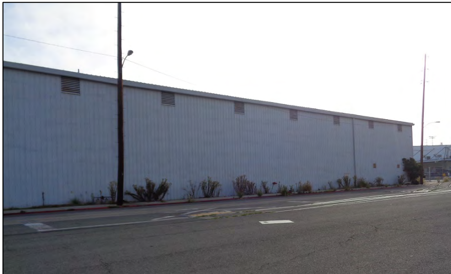
Photograph 2: west elevation, camera facing southwest. ICF, 2018.
