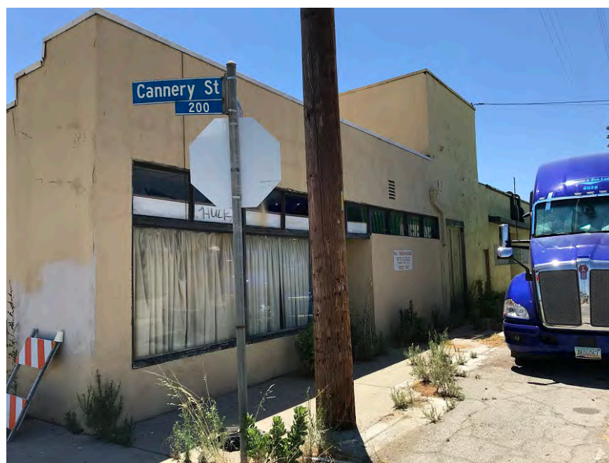
Figure 10-2. Nakamura Multi-Use Building, primary (west) elevation, camera facing southeast. ICF, 2020.
