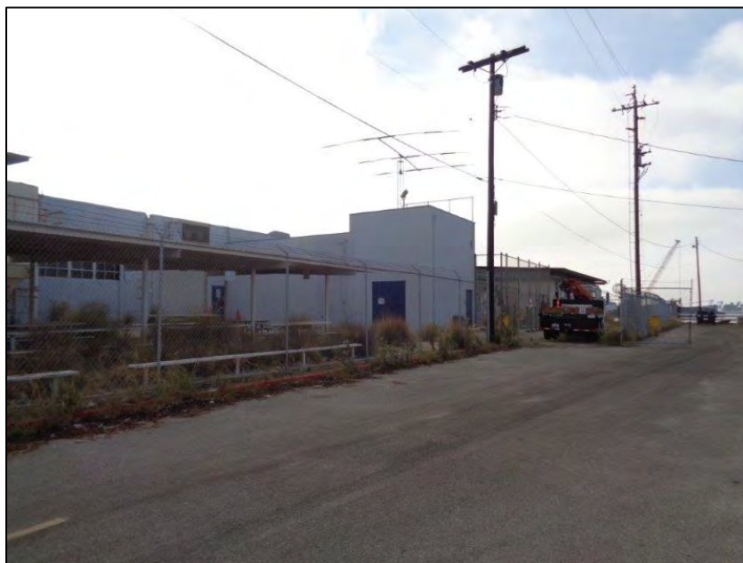
Figure 5-13. Star-Kist Plant No. 4, primary (west) elevation, overview of southwest corner of Plant (including volumes 7-9), camera facing southeast.
