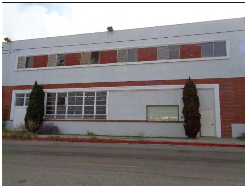
Figure 5-6. Star-Kist Plant No. 4, primary (west) elevation, detail of third volume from the north, north wing, camera facing east.
