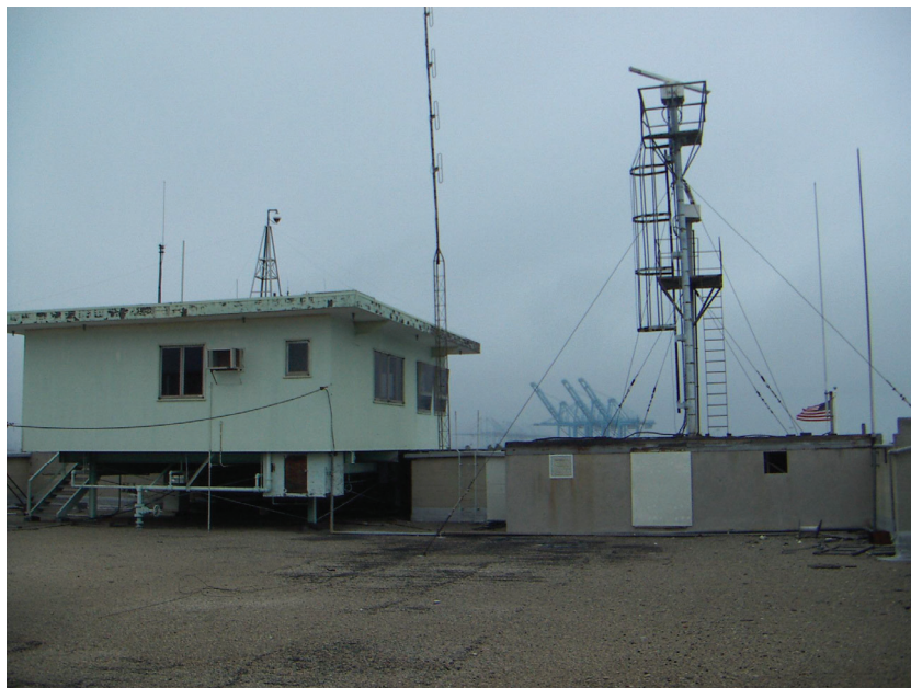
Figure 21 – Harbor Office and Equipment Penthouse on Roof
