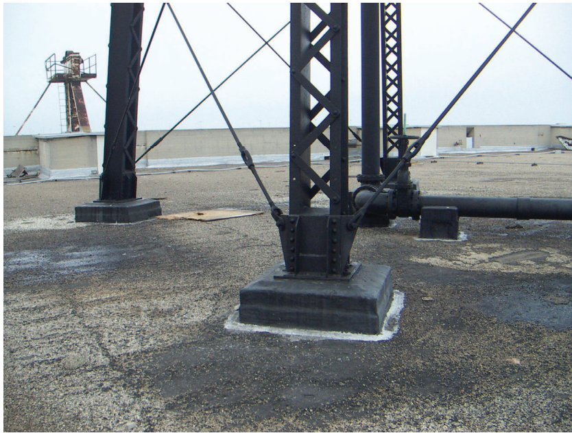
Figure 17 – Water Tank Base on Roof
