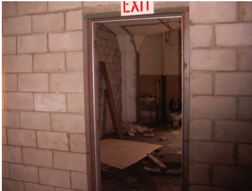
Figure 14 – CMU Infill Wall at Second Floor Restroom
