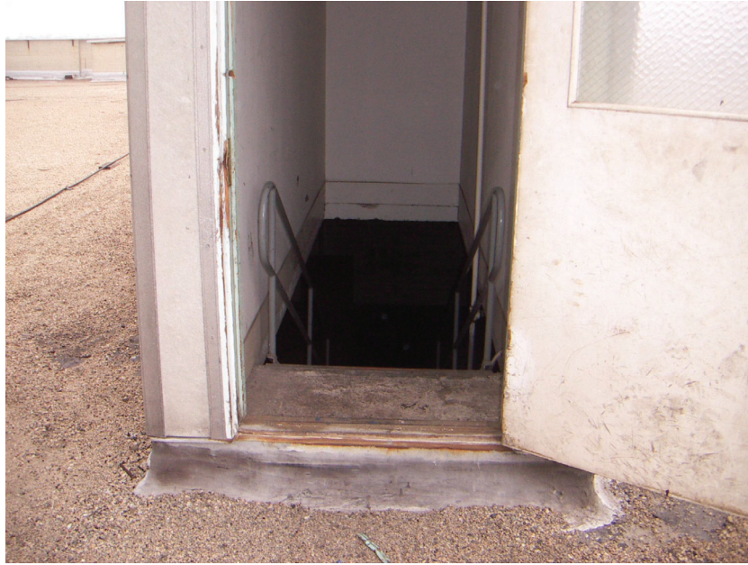
Figure 13 – Roof Opening at Southeast Corner for Stair
