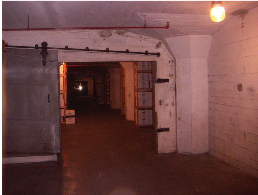
Figure 15 – Hallway Doorways At Upper Floor
