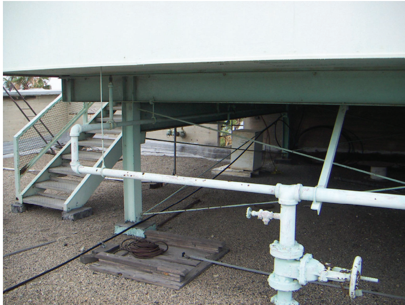
Figure 22 – Harbor Office Base on Roof
