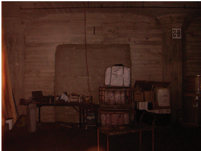
Figure 10 – Infilled Door Opening at First Floor
