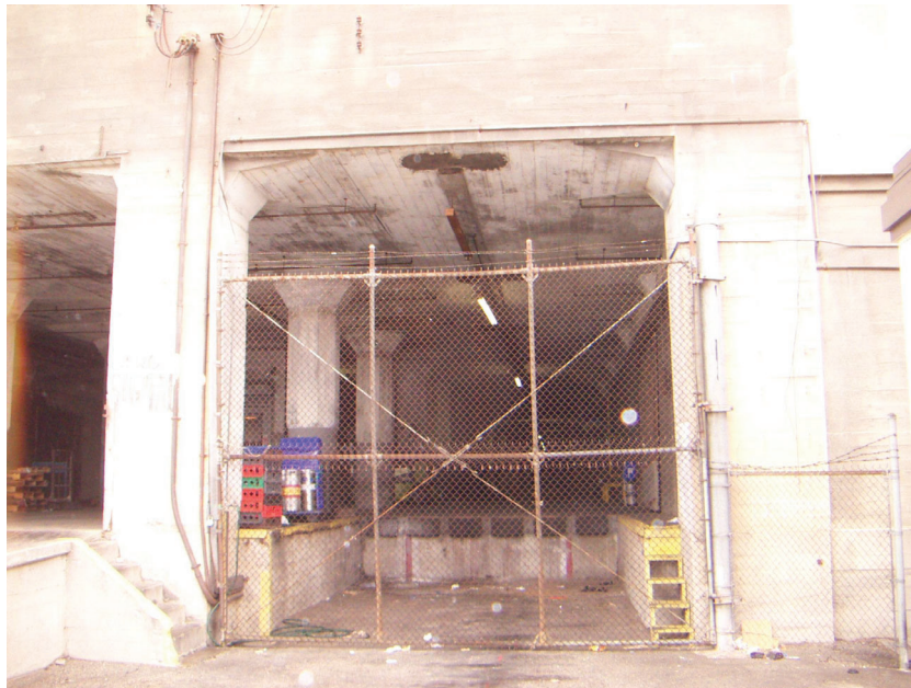
Figure 12 – Infilled West Railway at First Floor
