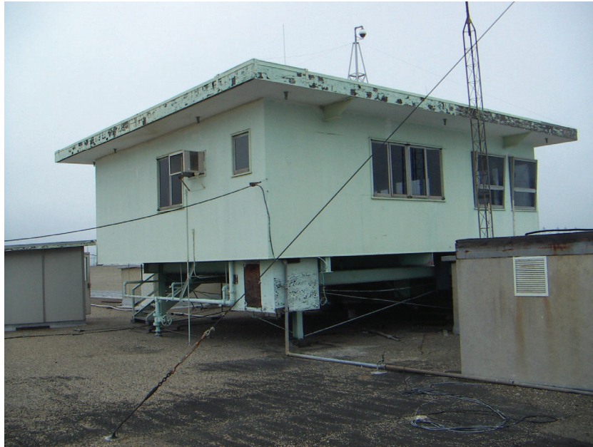
Figure 20 – Harbor Office on Roof
