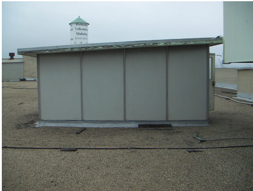
Figure 23 – Stair Penthouse on Roof
