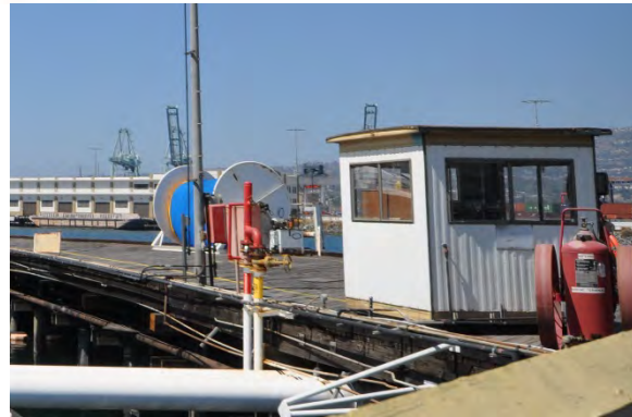
Figure 30: View looking southwest towards Wharf Building 4. (GPA, 2018)
