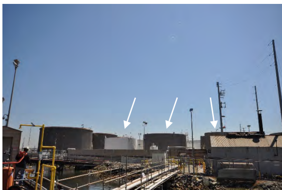
Figure 9: View looking northeast towards Tank Farm 2, arrows indicating westernmost tanks. (GPA, 2018)
