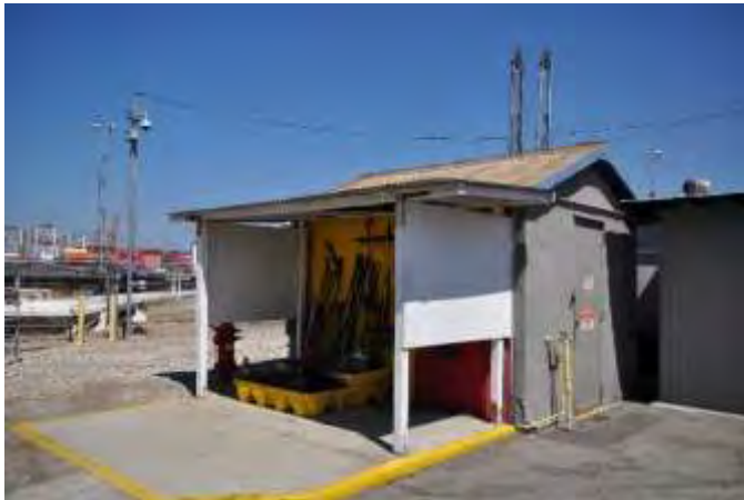
View looking NW at 5th of 8 pre-fabricated sheds, 8/6/18.
