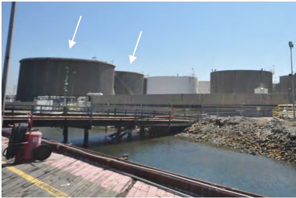
Figure 5: View looking northeast towards Tank Farm 1, arrows indicating two westernmost tanks. (GPA, 2018)
