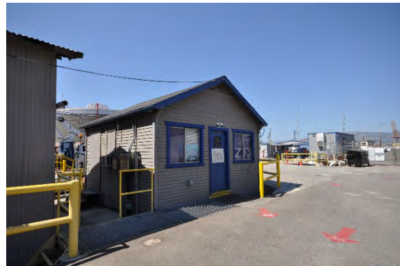
Figure 16: View looking southeast towards Office 3. (GPA, 2018)
