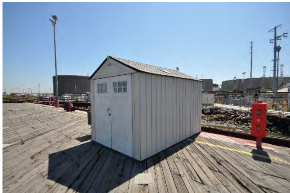
Figure 27: View looking northeast towards Wharf Building 1. (GPA, 2018)
