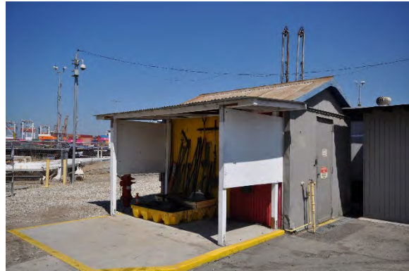
Figure 18: View looking northwest towards the fifth of eight pre-fabricated sheds. Corrugated metal shed. (GPA, 2018)
