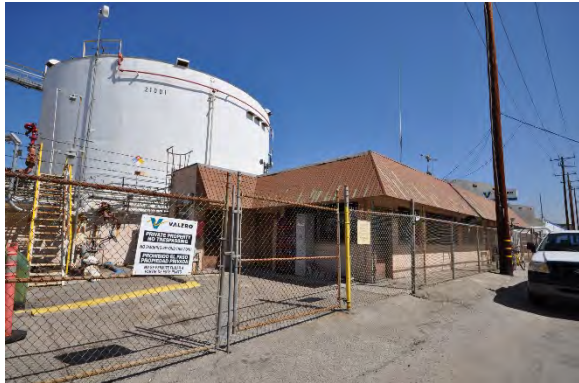
Figure 21: View looking northwest towards Office 4. (GPA, 2018)
