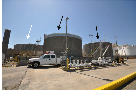
Figure 14: View looking east towards Tank Farm 3, arrows indicating tanks in Tank Farm 3. Black arrows indicating tanks in secondary dike wall. (GPA, 2018)
