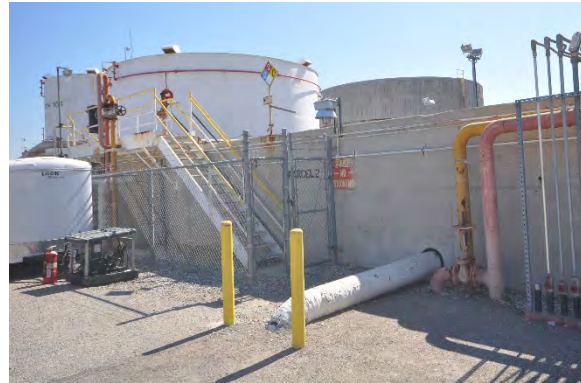
Figure 22: View looking east towards Tank Farm 4 and access stair. (GPA, 2018)
