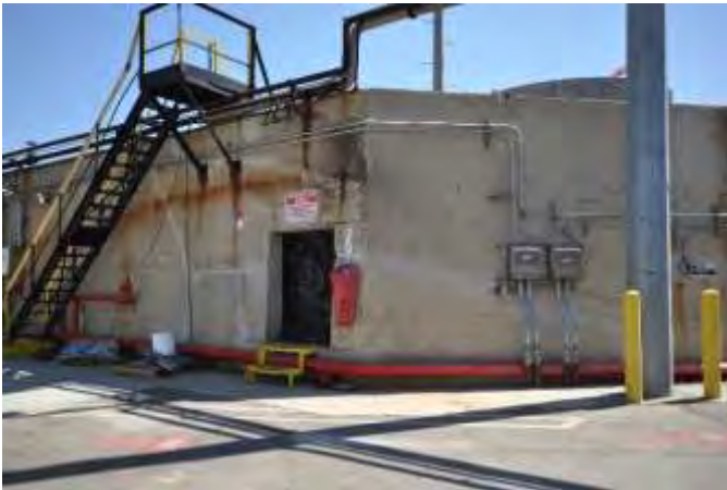
View looking NE at Tank Farm 2 dike wall entrance, 8/6/18
