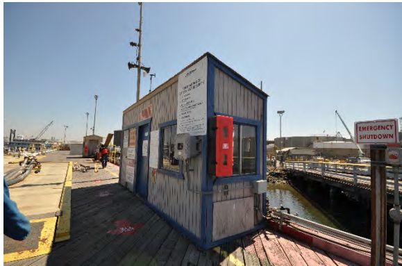
Figure 29: View looking northeast towards Wharf Building 3. (GPA, 2018)
