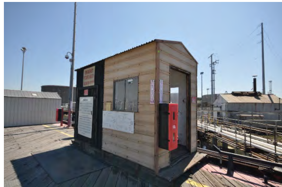
Figure 28: View looking northeast towards Wharf Building 2. (GPA, 2018)
