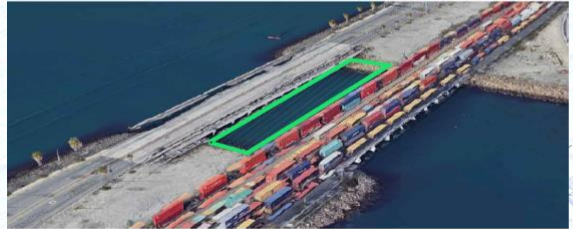
BRIDGE OBLIQUE VIEW
