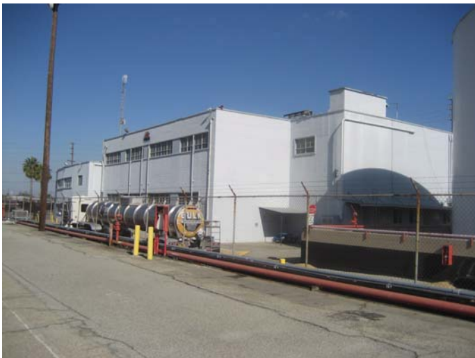
Office Building by Berth 187
