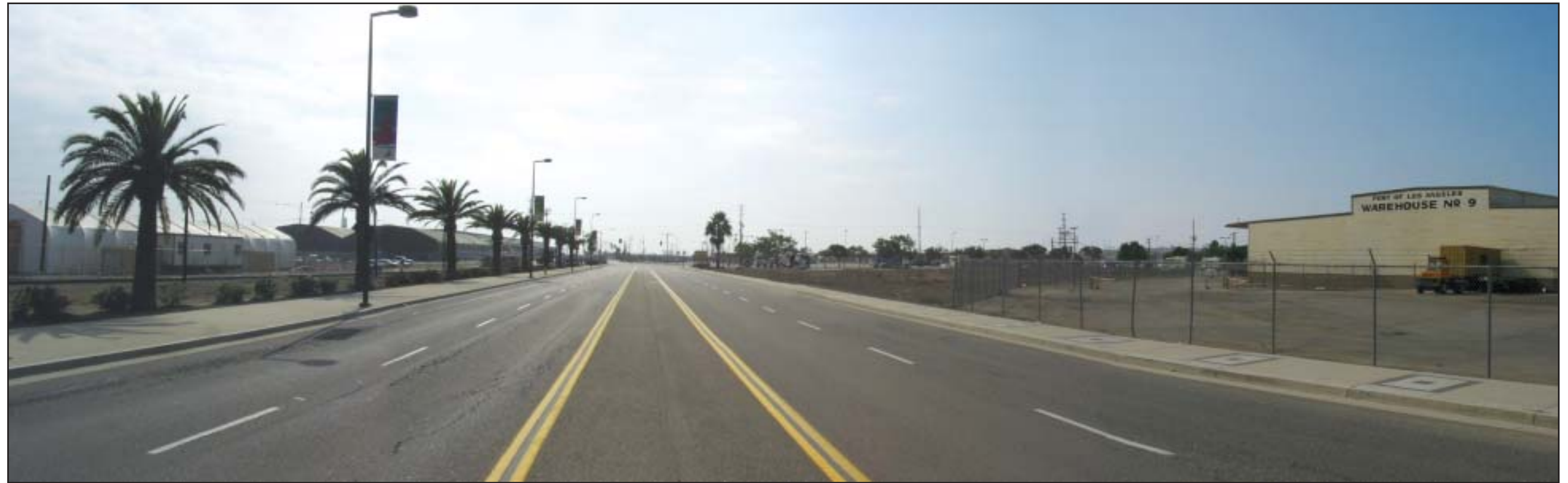
Photo A : View from Miner Street.
