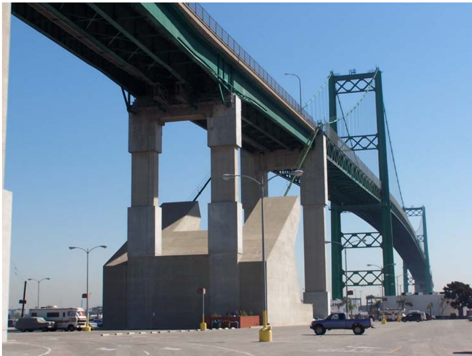
Vincent Thomas Bridge, 2001, Los Angeles Public Library photo archive
