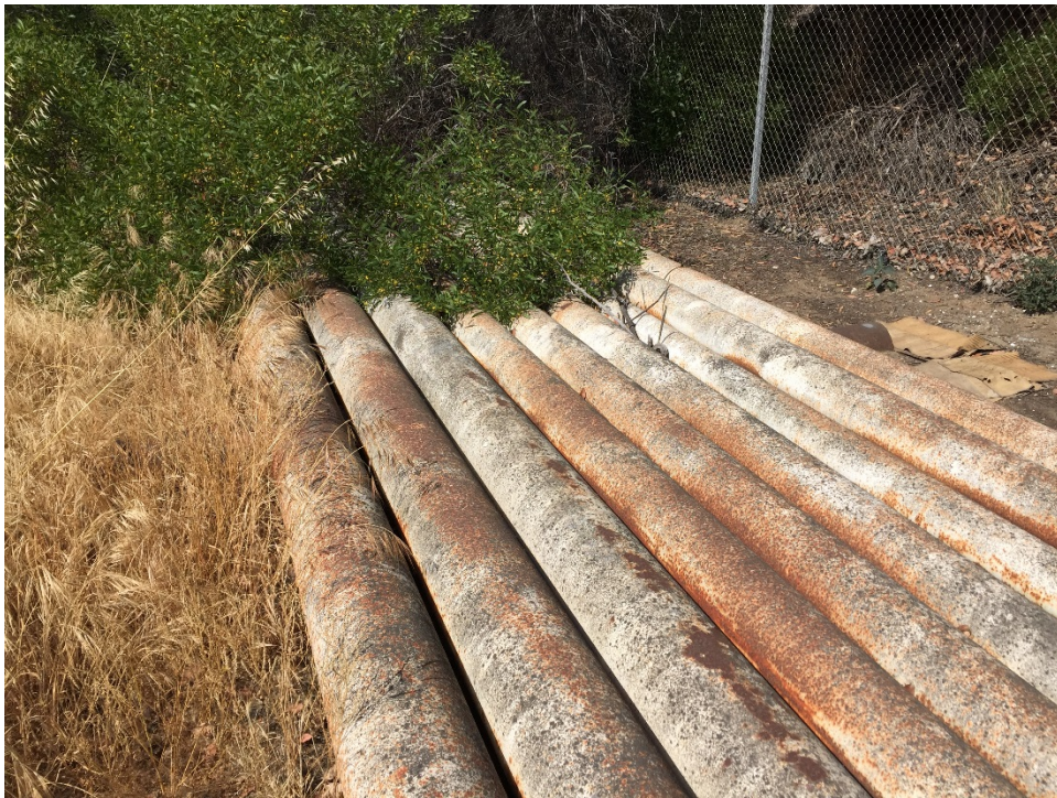
Photo 26 – Pipelines extending along the northwestern fence line, adjoining the Harbor Freeway.
