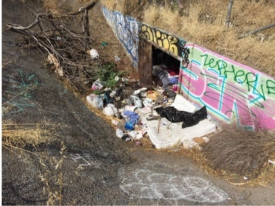
Photo 39 – Another culvert on the northern portion of the Property.
