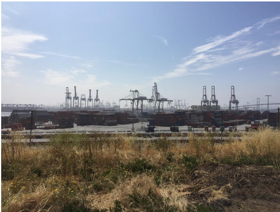
Photo 36 – Port facilities to the east of the Property.
