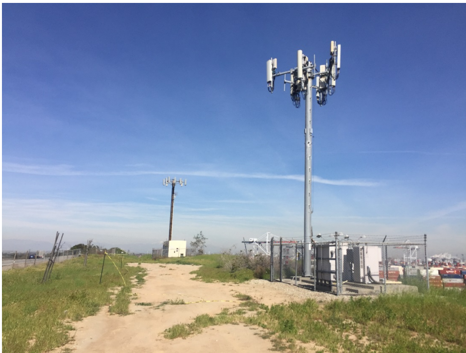
Photo 6 – Cellular towers and associated electrical equipment located on the central portion of the Property.
