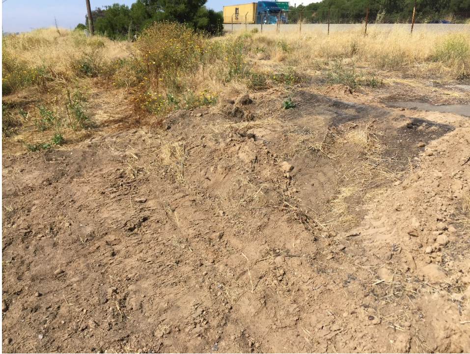
Photo 37 – Area of cleared vegetation with discolored soil on the northern end of the Property.
