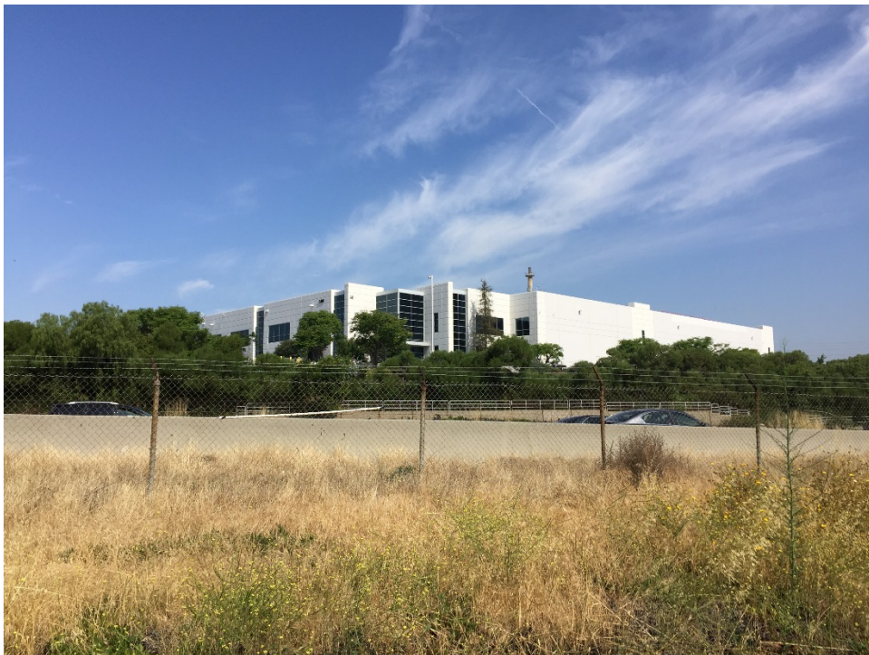
Photo 32 – View to the north of the Property.
