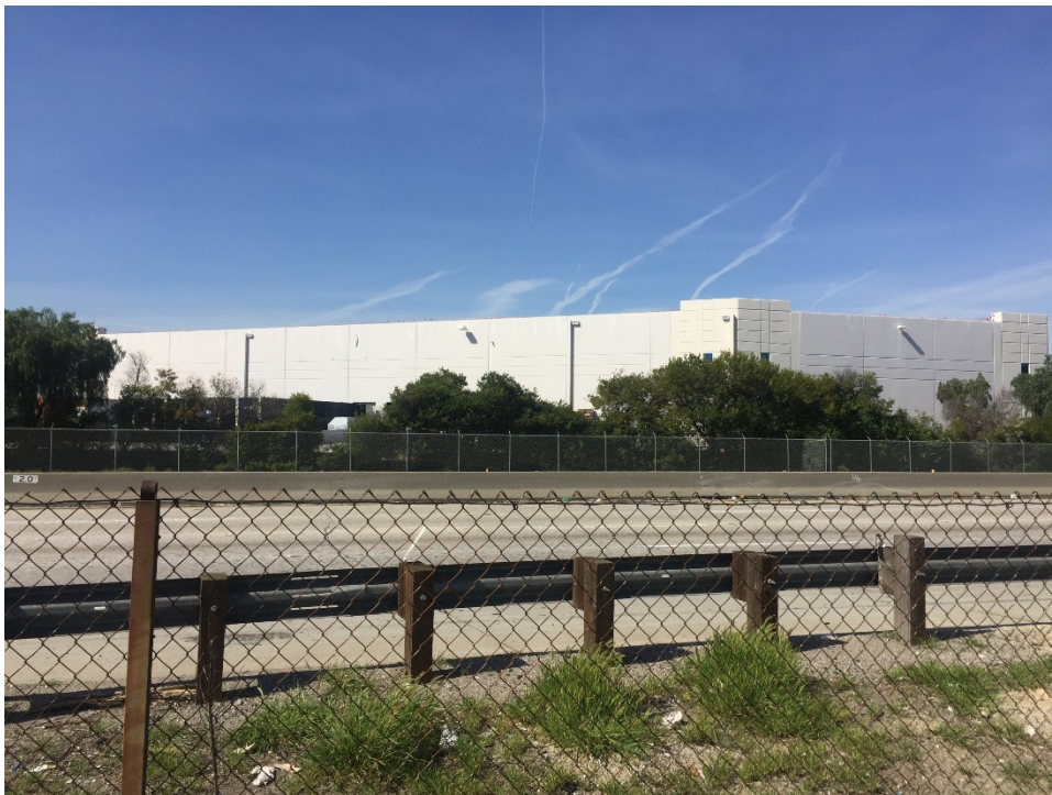
Photo 4 – View from the central portion of the Property looking across the adjoining Harbor Freeway to the north.
