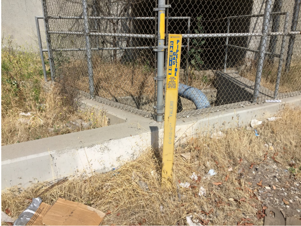
Photo 45 – Gas pipeline marker and culvert just outside the northern end of the Property.
