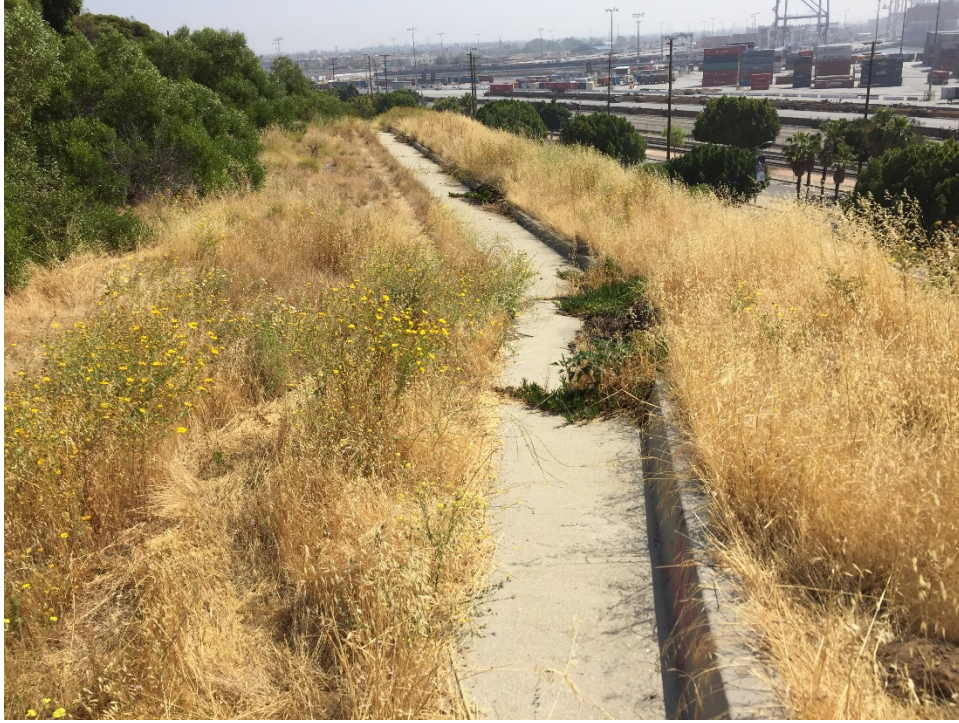
Photo 25 – Curb and gutter remnants on the central-western portion of the Property.
