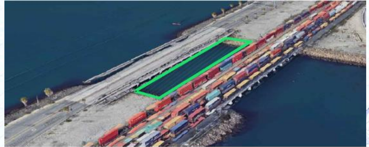
BRIDGE OBLIQUE VIEW
