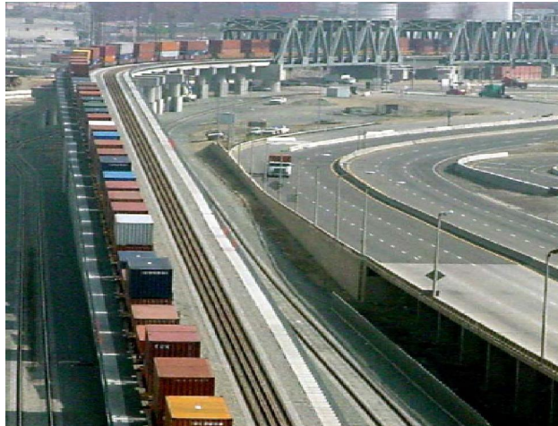
Figure 1-10. Assembled Container Train.
