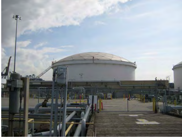
Photograph 4. View of storage tank M-10, view southeast.
