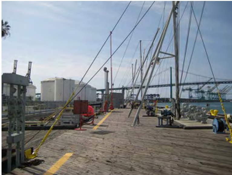
Photograph 1. Overview of timber wharf, Berths 167-169, view to the south.
