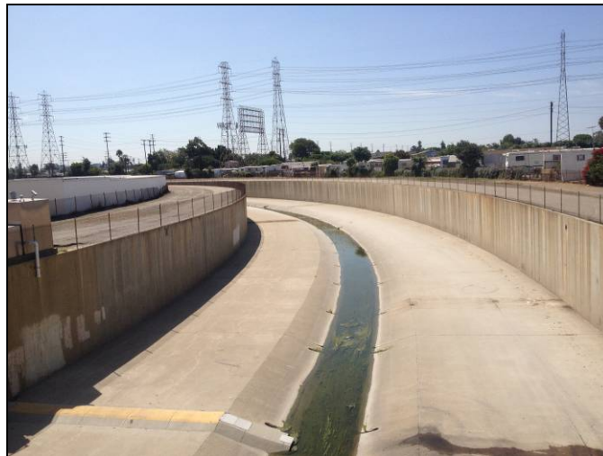
Figure 2-3. Dominguez Channel Monitoring Location (DC)
