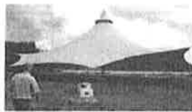
Exhibition hall - 1982 Port-Gentil, Gabon - Preconstraint 1302 Tensile resistance after 18 years: Warp 86% - Weft 76%
