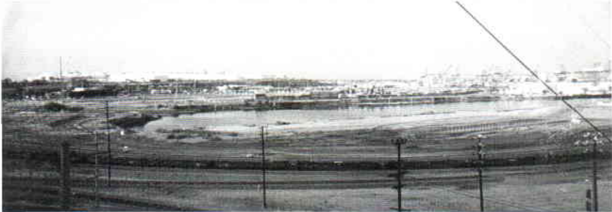
Panoramic View from Intersection of Summerland, MacArthur and Elberon Avenues, early 2002
