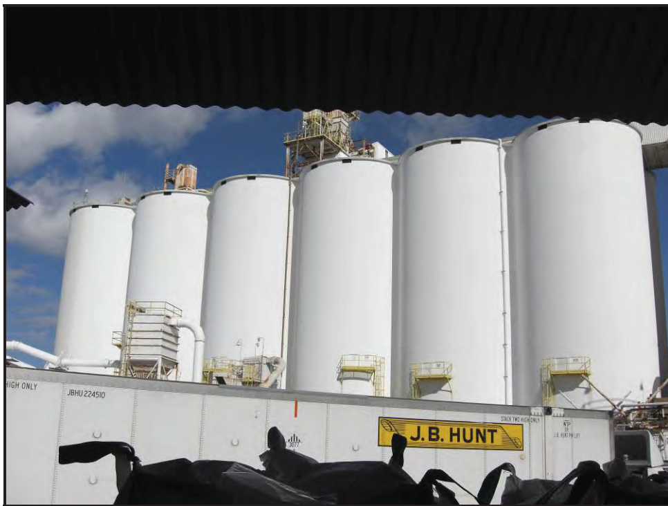
Looking northeast at a grouping of non-historic period storage silos.
