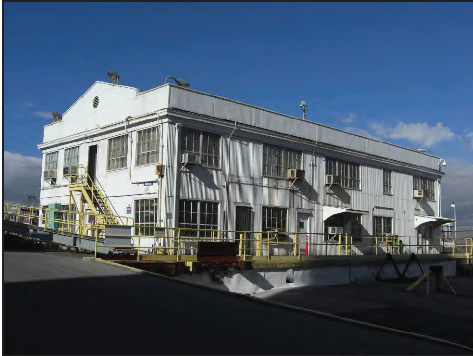
Looking northwest at Wharf Office Building.
