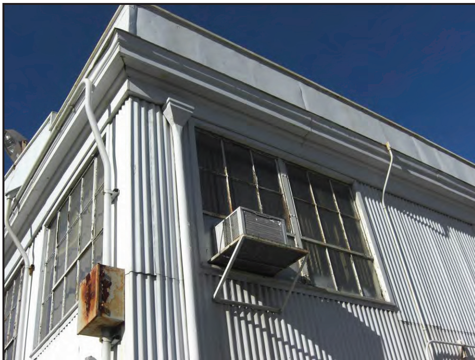
Detail of south east wall of Warehouse Office Building.
