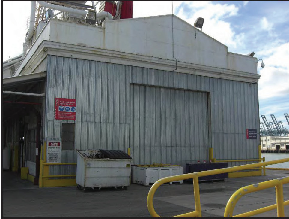
Looking southwest at Warehouse Building.
