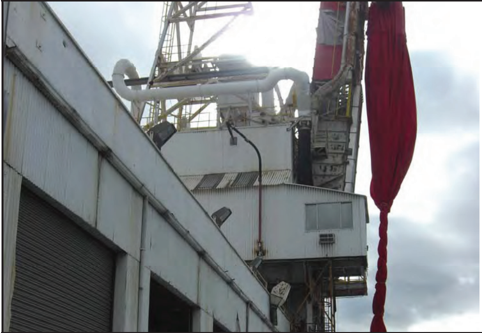
Looking southeast at detail of non-historic period addition to Warehouse Building.
