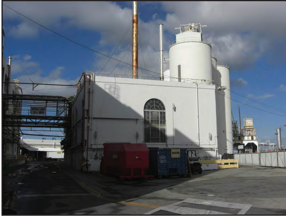
Looking west at the Power Plant.
