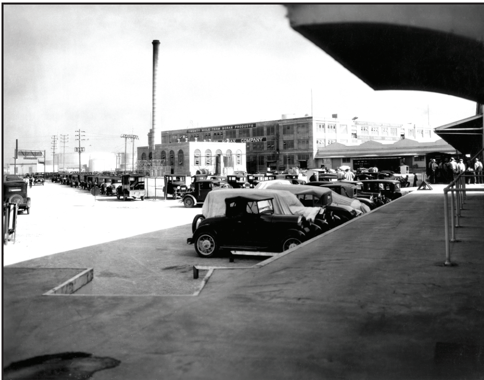
Historic-period photograph looking southeast from loading dock area of Warehouse Building.
