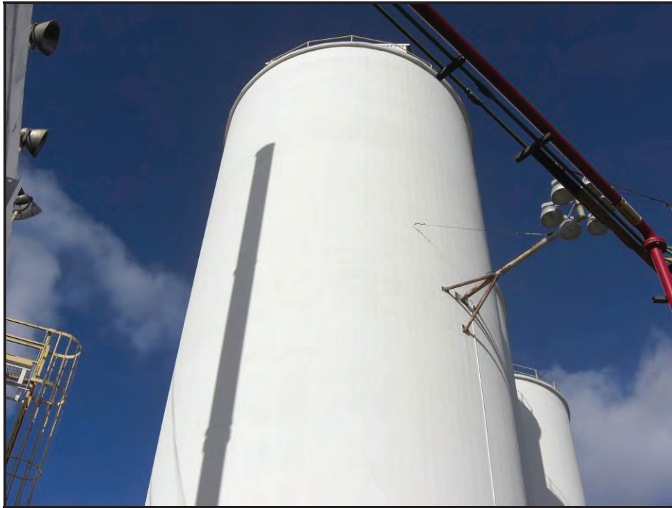
Looking northwest at a non-historic period storage silo.
