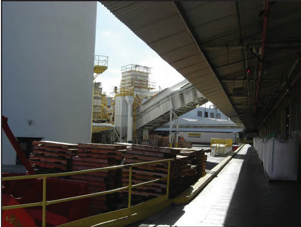
Looking southeast from loading dock area of Warehouse Building.
