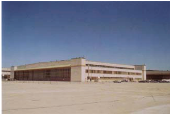
Figure 31. Building 40 (Seaplane Hangar), 2004
