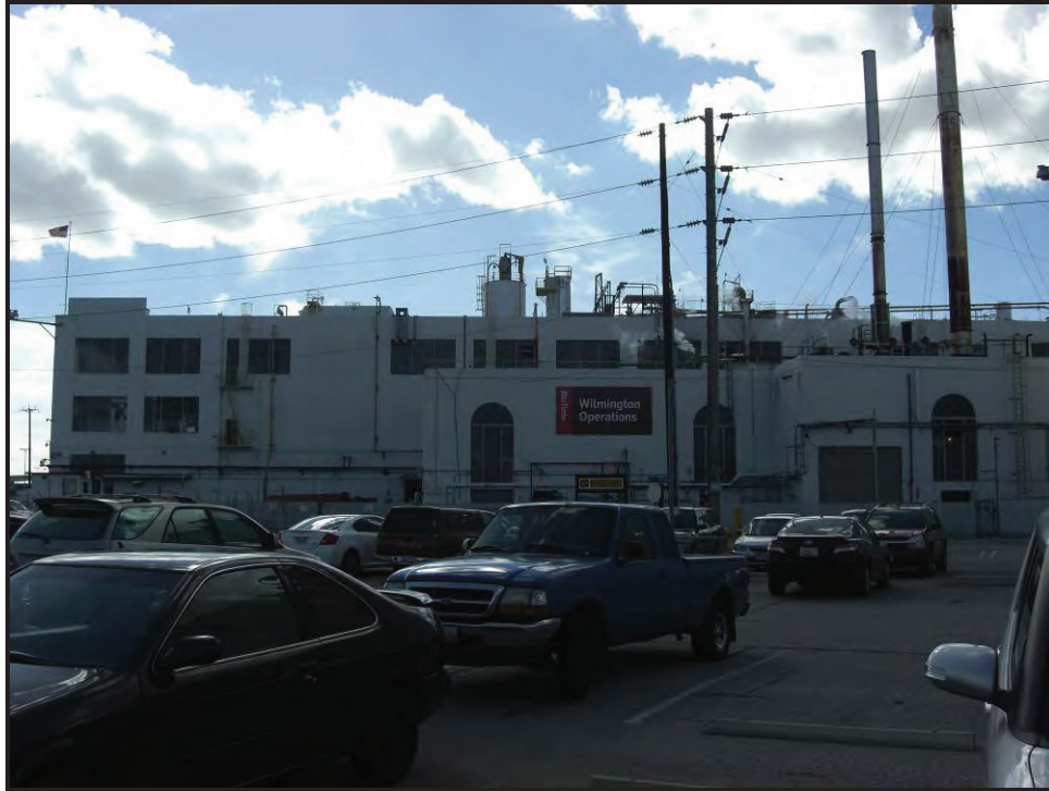
Looking south at the north elevation of the Refinery Building with Power Plant in foreground.
