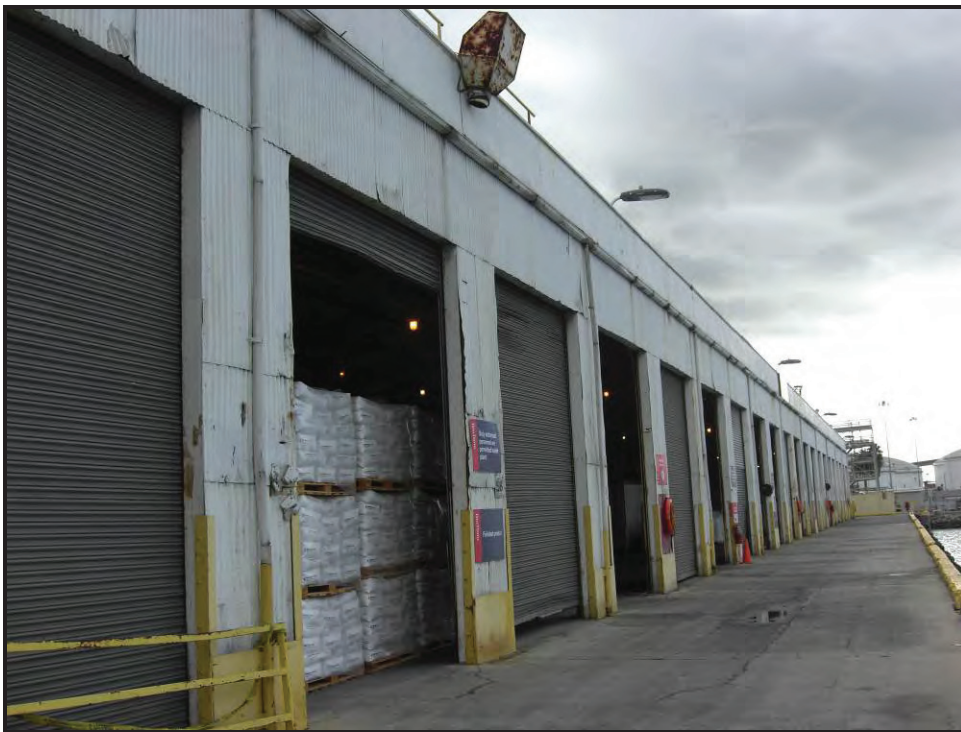
Looking southeast at Warehouse Building.
