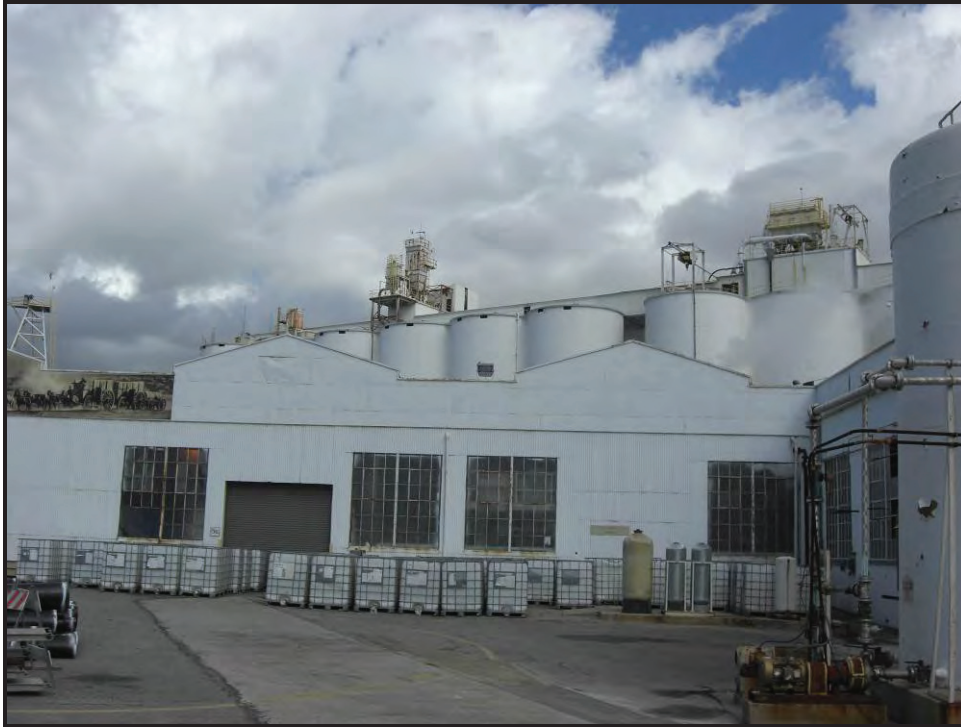
Looking north at the south elevation of the Connecting Building.
