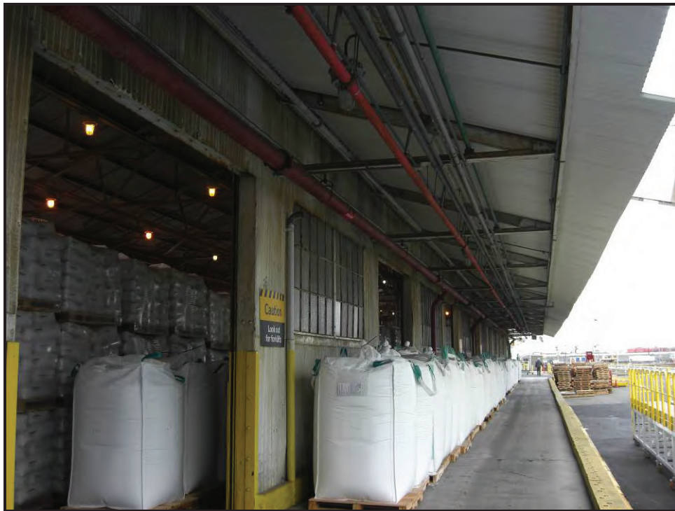
Looking northwest at Warehouse Building.
