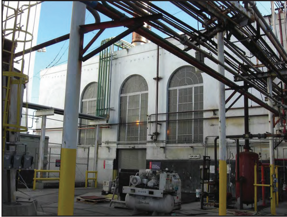
Looking east at alterations and non-historic period equipment added to Power Plant.
