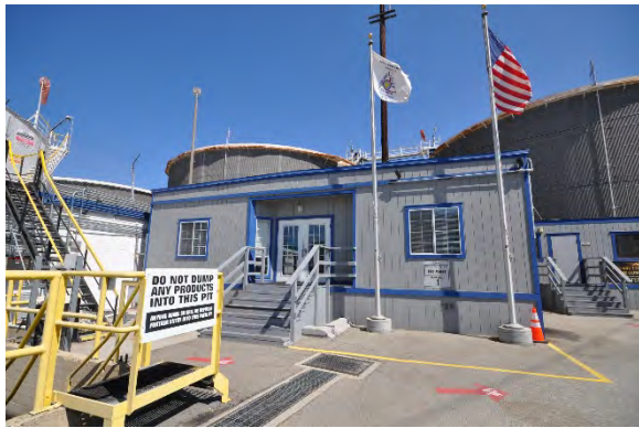
Figure 7: View looking northeast towards Office 1, the larger of the two prefabricated office buildings outside the dike wall. (GPA, 2018)
