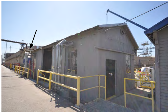
Figure 15: View looking southeast towards Storage Building 1 and Gabled Shed (shown with arrow). (GPA, 2018)
