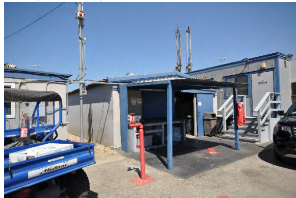
Figure 20: View looking northwest towards the seventh and eighth of eight pre-fabricated sheds. (GPA, 2018)
