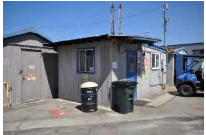
View looking NW at 5th and 6th of 8 pre-fabricated sheds, 8/6/18.
