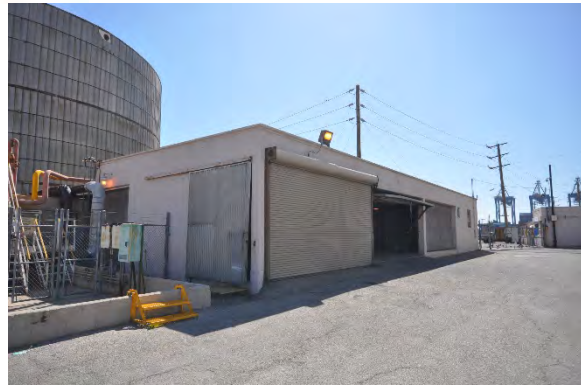
Figure 24: View looking east towards Storage Building 2. (GPA, 2018)
