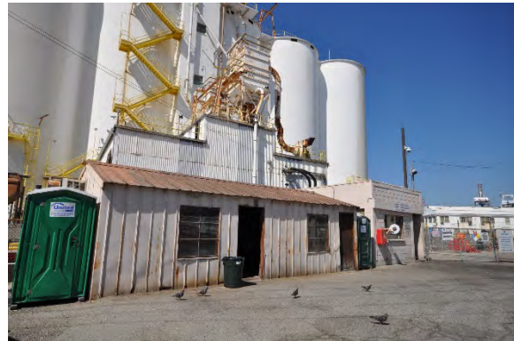
Figure 26: View looking southwest towards Office 5. (GPA, 2018)
