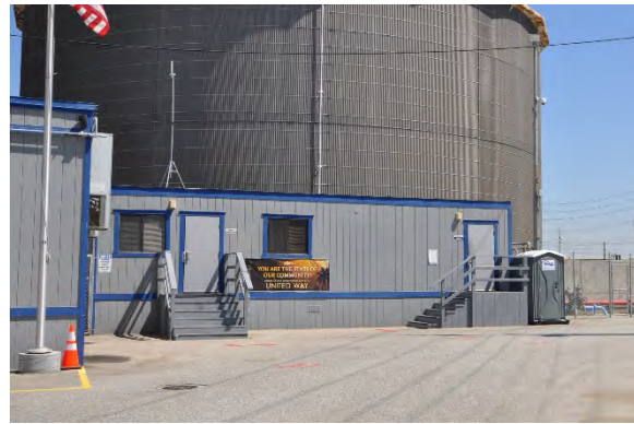
Figure 8: View looking northeast towards Office 2, the smaller of the two prefabricated office buildings outside the dike wall. (GPA, 2018)
