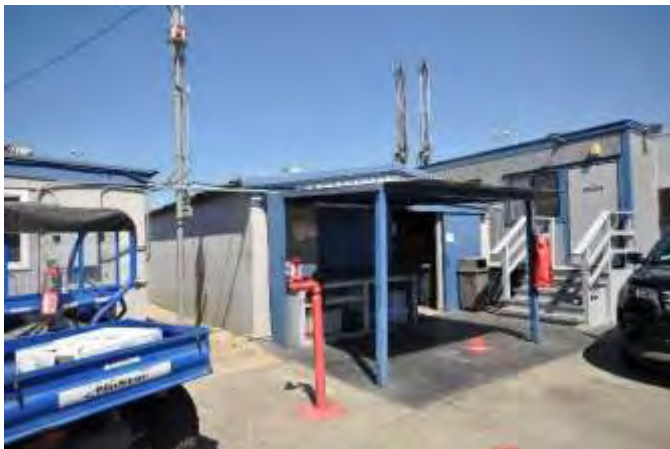
View looking NW at 7th and 8th of 8 pre-fabricated sheds, 8/6/18.
