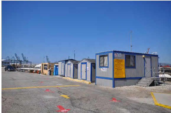
Figure 17: View looking northwest towards four of eight pre-fabricated sheds. (GPA, 2018)
