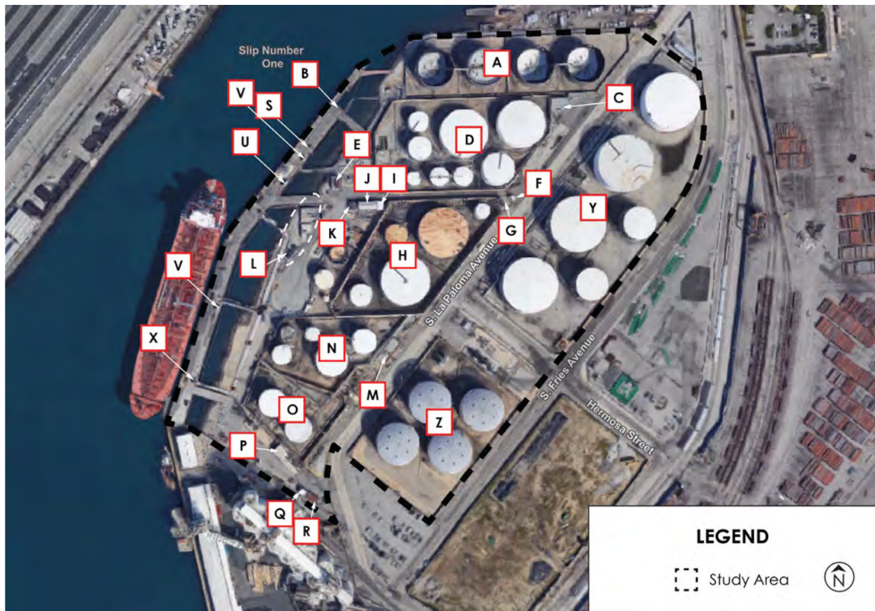
Figure 4: Buildings and Structures on Berths 163 and 164. Base image courtesy of Google Maps.
