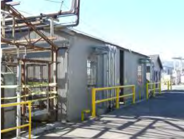
2014 Applied Earthworks photo, view looking west (gabled shed not present).
