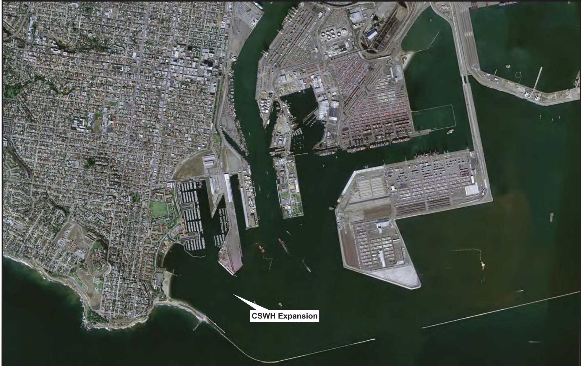
Figure 3.1-4 Cabrillo Shallow Water Habitat Expansion Site – Aerial View
