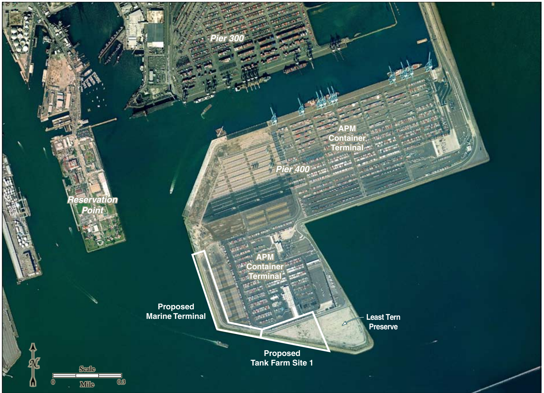
Figure 3.1-1. Aerial Photograph of Pier 400, taken in February 2004
