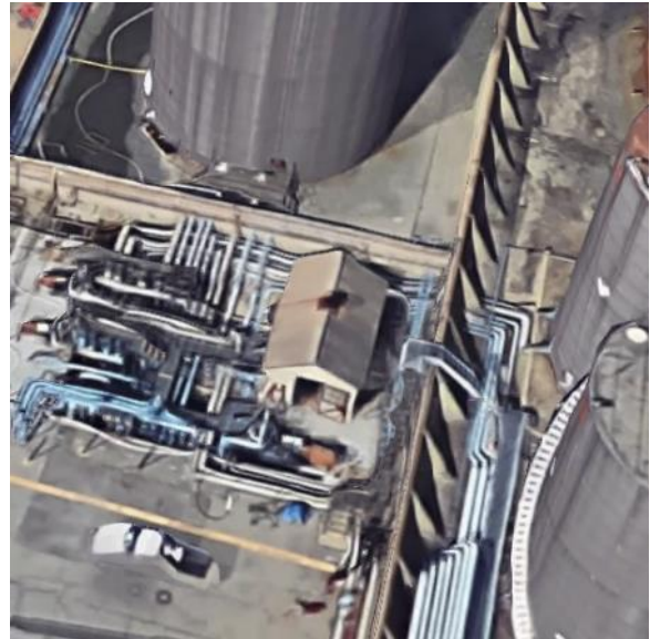
Figure 17: Aerial view of Pump House 2, view looking west. Google Maps.
