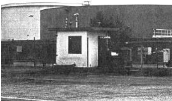
Figure 14: Gate House as it appeared in 2000. Jones & Stokes.
