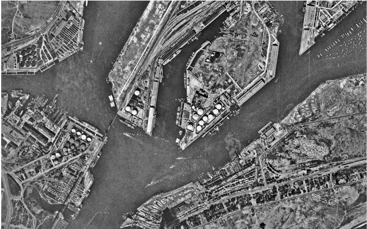
Figure 43: Terminal at Berth 150-151 and its surroundings in 1927. Terminal indicated with yellow ellipse. Historic aerial courtesy of USCB Library.
