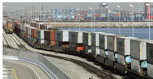
Photograph 3. The Port's rail infrastructure consists of more than 65 miles of on-dock track for building and sorting double-stack trains. The average train is made up of 30 double-stack cars, eliminating approximately 400 truck trips and related air pollution while optimizing the movement of cargo.
