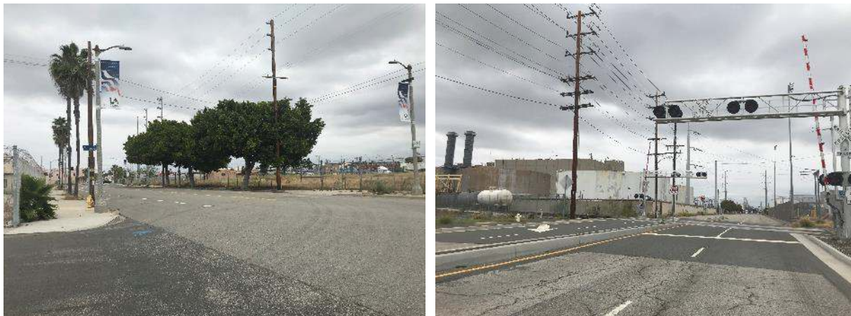
Photograph 2. The Project site includes segments of the Fries Avenue, Avalon Boulevard (left), and "A" Street. Avalon Boulevard and Fries Avenue cross the Union Pacific railroad tracks and right-of-way (right). "A" Street is located north of the railroad tracks and provides a connection between Fries Avenue and Avalon Boulevard.
