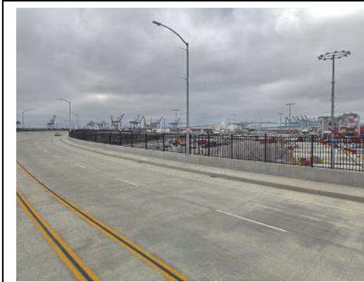
Photograph 4. The South Wilmington Grade Separation was opened in April 2015 and provides an overpass with four lanes of traffic (35 miles per hour) as well as pedestrian sidewalks.
