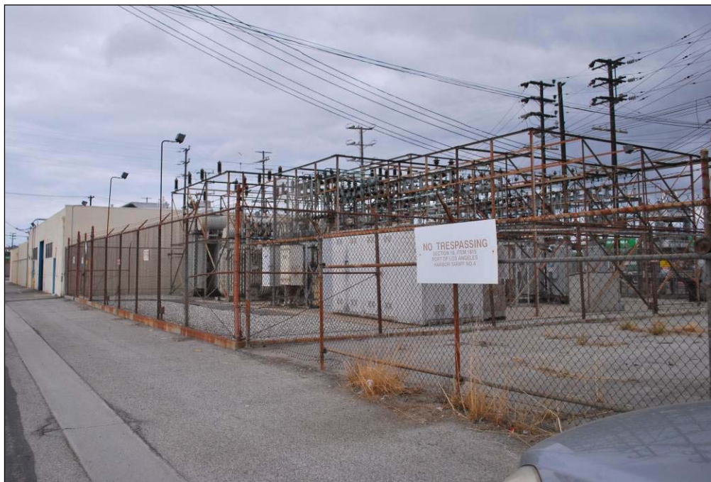
Figure 23. Overview of Distribution Station 121; view facing northwest, 2014.
