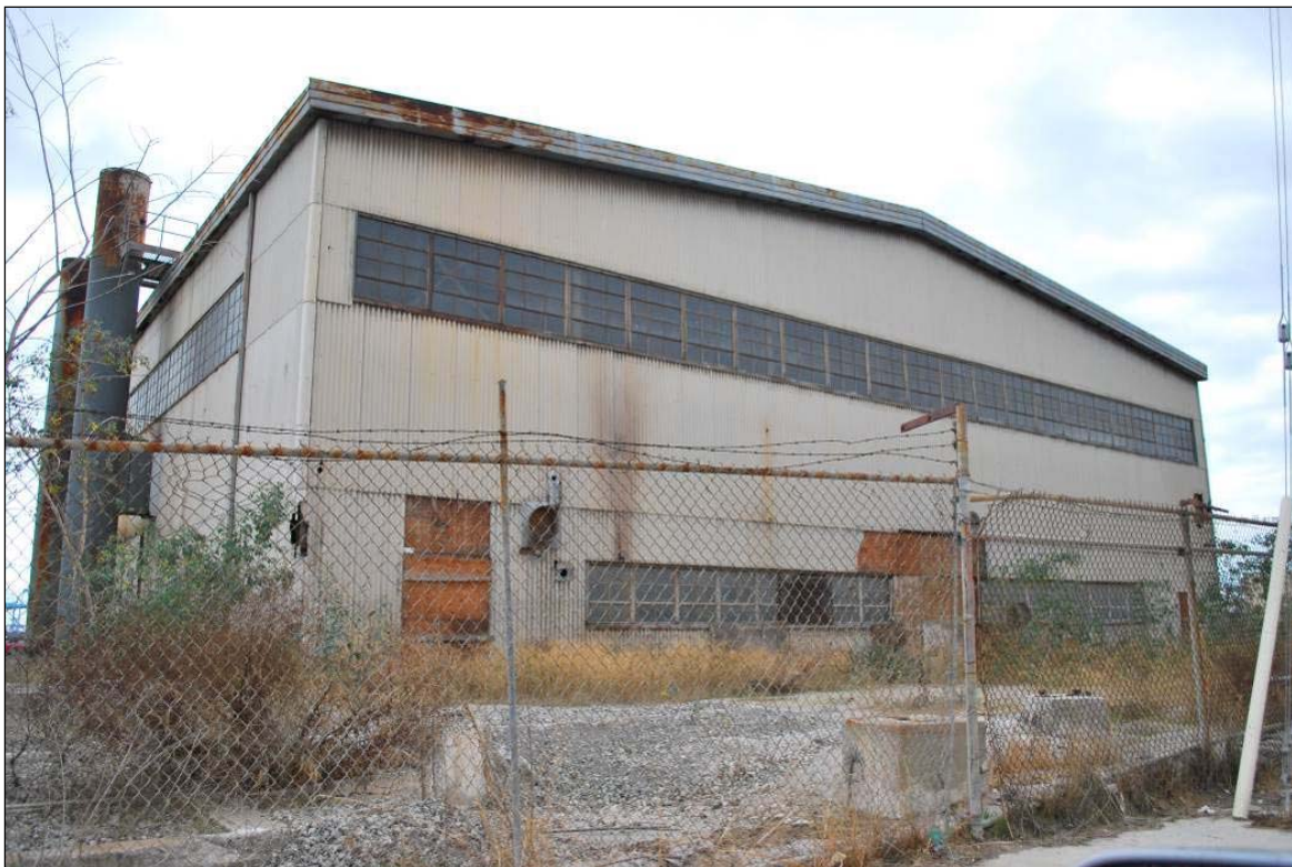
Figure 18. Rear (north) of property where steam generating plant; view facing southwest, 2014.
