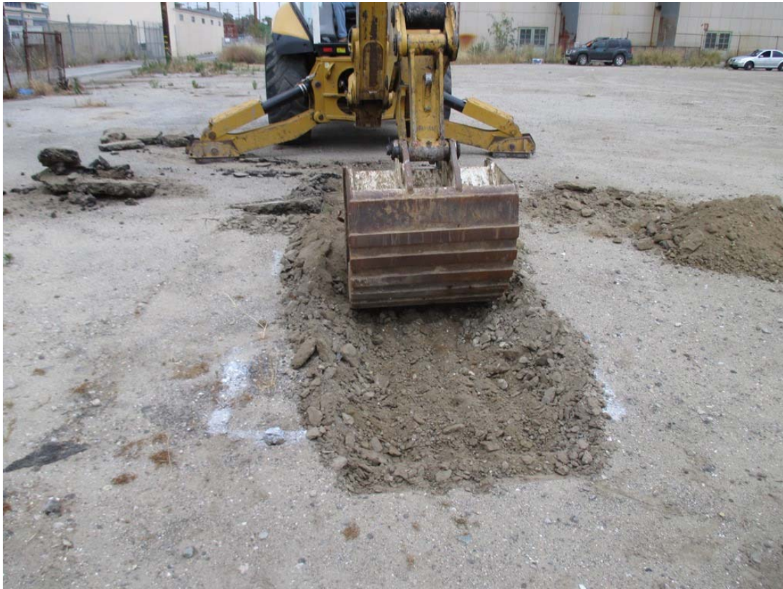
Figure 15. Backhoe excavating MTR 1011; view facing northeast.
