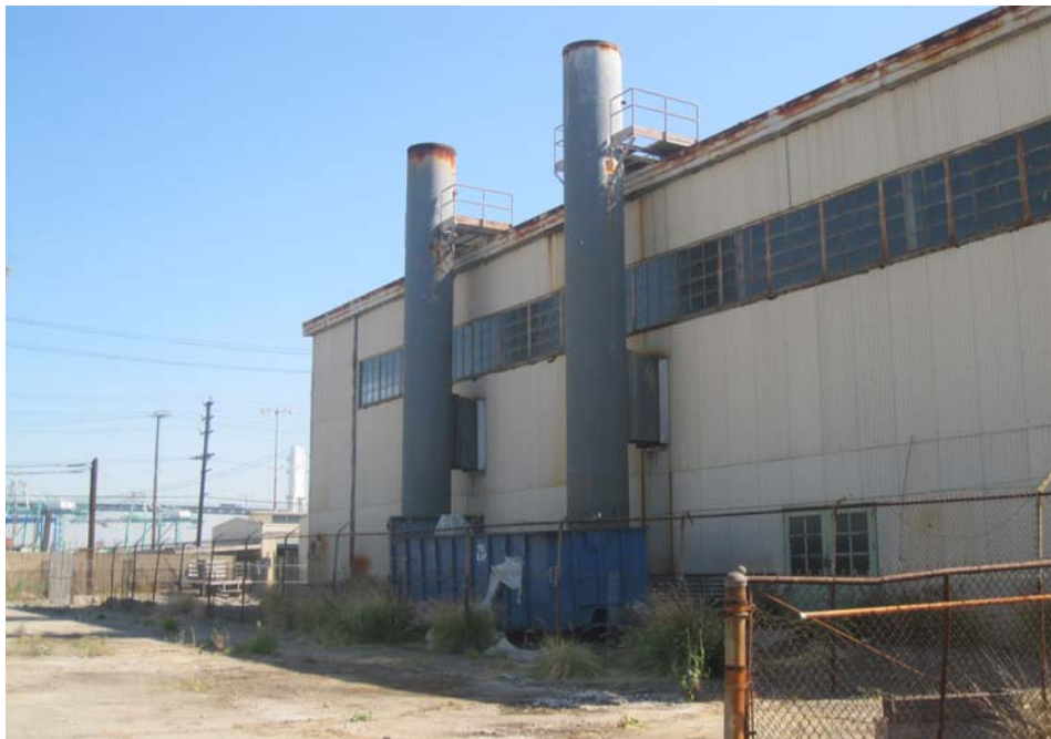
Photograph 4. Canner's Steam Company Plant, Facing Northeast
