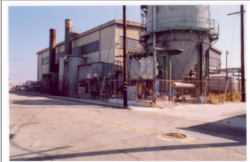
Canner's Steam Company Plant, Facing Southwest
