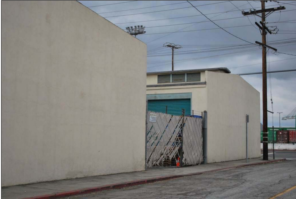
Figure 21. Front (east) of the Net Shed Storage Complex; view facing northwest, 2014.
