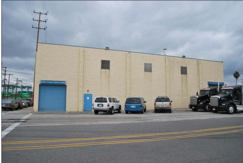
Figure 20. Overview of the Pilot Plant; view facing north, 2014.
