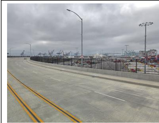
Photograph 5. The South Wilmington Grade Separation was opened in April 2015 and provides an overpass with four lanes of traffic (35 miles per hour) as well as pedestrian sidewalks.
