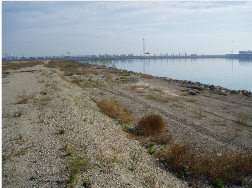
Berth 306, note channel cut by runoff to left side.
