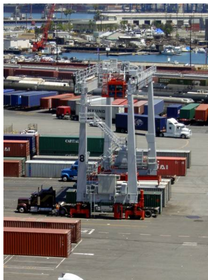
Figure 4.8: Rubber Tired Gantry Crane
