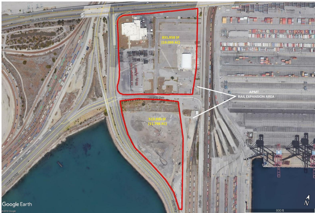
Figure 2 – Site Boundary: Pacific Crane Maintenance Company
