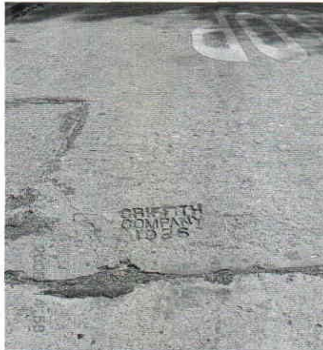
South View - 400 Block of Elberon Avenue, Black Hill
