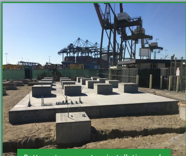
Battery storage system installation pads
