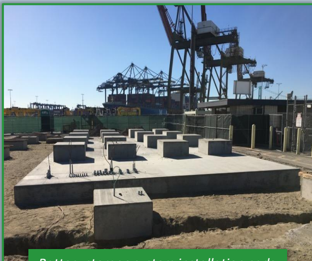
Battery storage system installation pads
