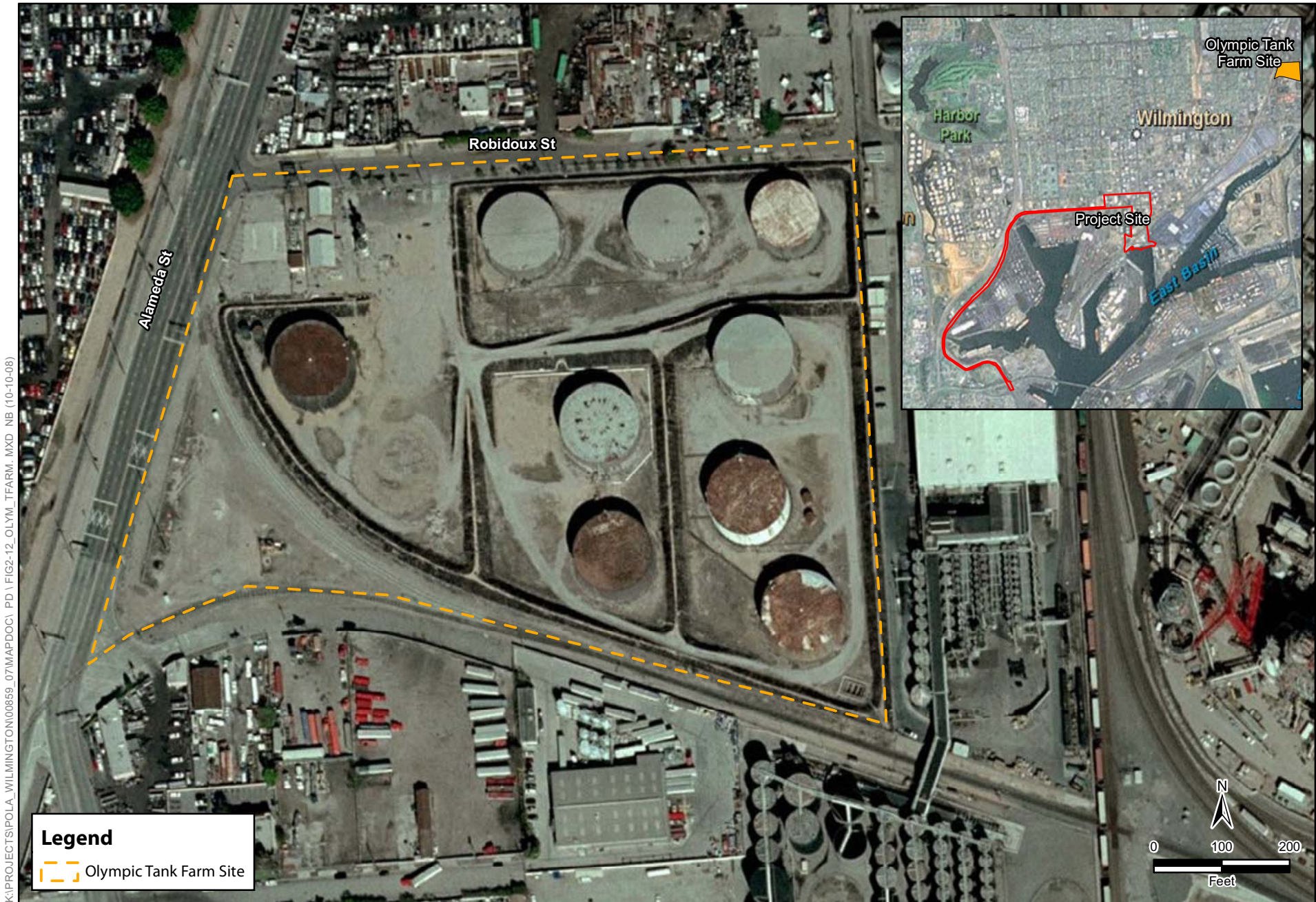
Figure 2-12 Aerial View of Olympic Tank Farm Wilmington Waterfront Development Project
