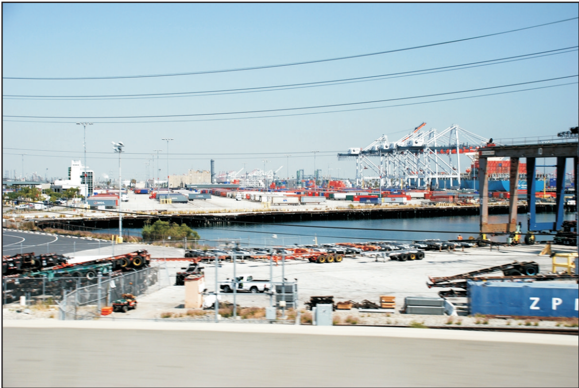
KOP F Existing Viewshed Conditions - Northbound Travel Lanes of I-110 near the C Street offramp, View Direction East
