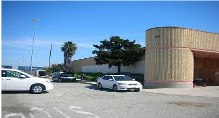
Figure 2-4 North Side of Navy Commissary Building 390 Navy Way
