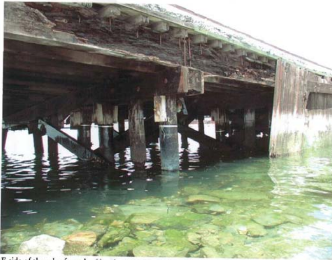
Site 1 pool and wharf pilings
