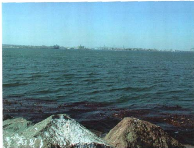
Site 3, western breakwater
