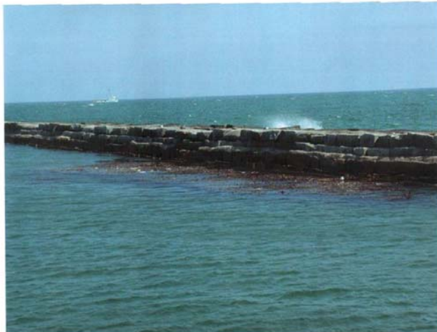
Site 3, western breakwater from end of Fishermen's Pier
