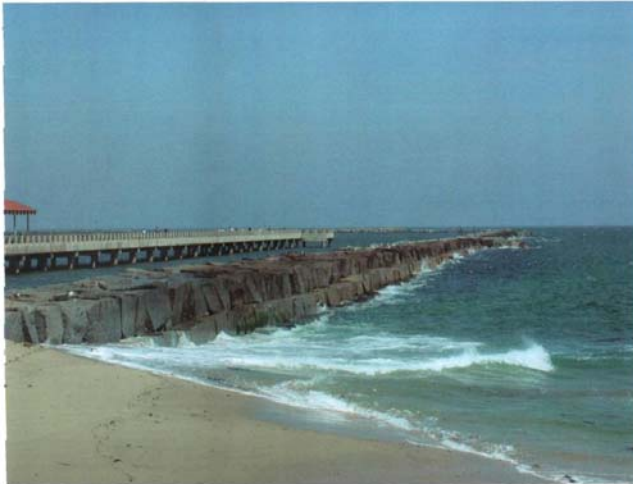
Photo of the W breakwater looking E from access to Fishermen's Pier. Sand has filled in from the County beach on this ocean side of the breakwater. A groin was built into the ocean from the breakwater to facilitate sand capture for the beach. Evidently the County beach had diminished sand for a time. The Fishermen's Pier is the concrete pier extending from left of photo to about photo center.
