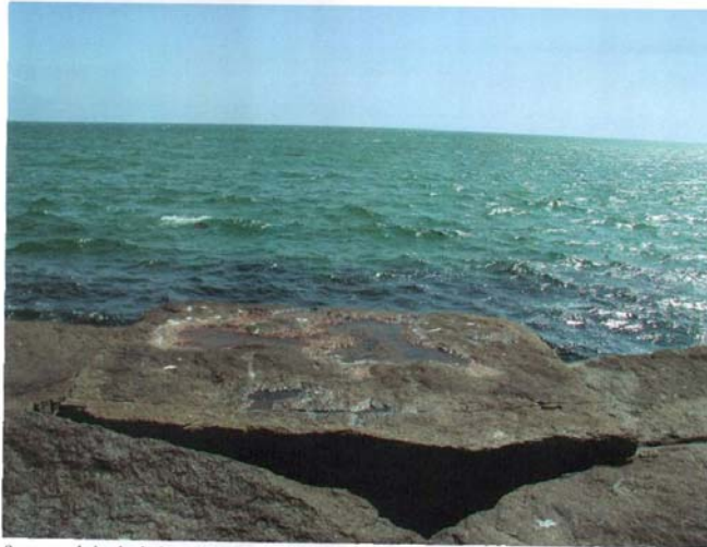
Site 3, western breakwater
