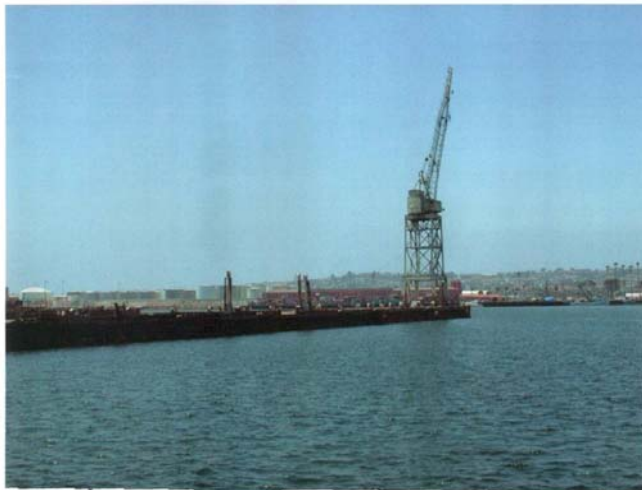
South dock at fill area of berths 243-245
