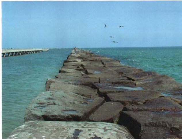
Site 3, western breakwater
