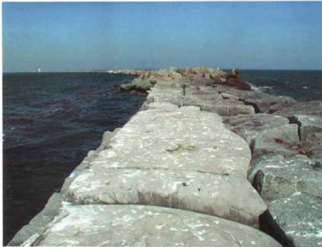
Site 3, western breakwater
