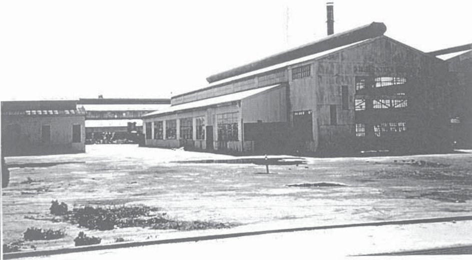
Photograph 2. Shed-roofed, metal-sided extension
