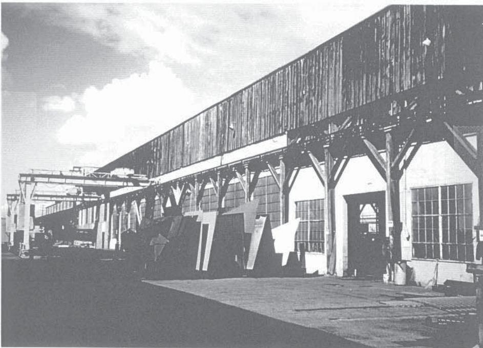
Photograph 2. West elevation showing wood trusses
