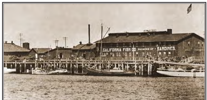
California Fish Company's first building, destroyed by fire in 1914 (Queenan 1983).
