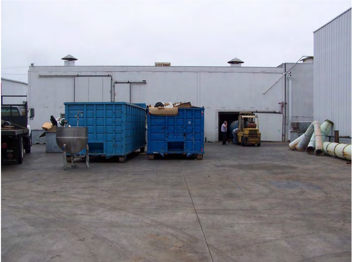
Photograph 1. California Marine Buildings, facing south. 05.02.2006.
