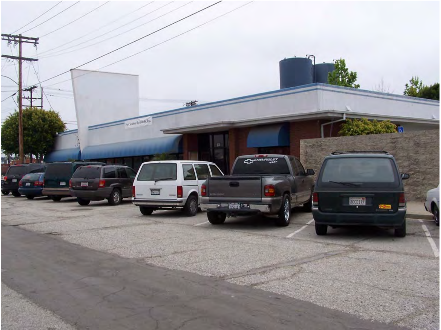
Photograph 5. Chicken of the Sea Plant main office, facing southwest. 05/02/2006.
