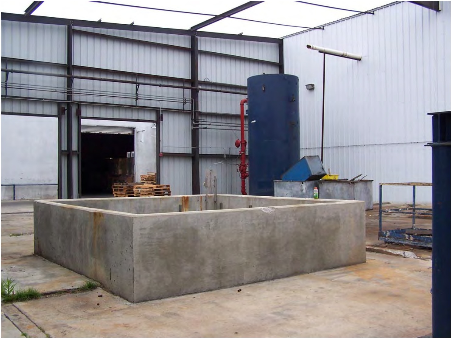
Photograph 3. Fish Oil Tanks. 05.02.2006.
