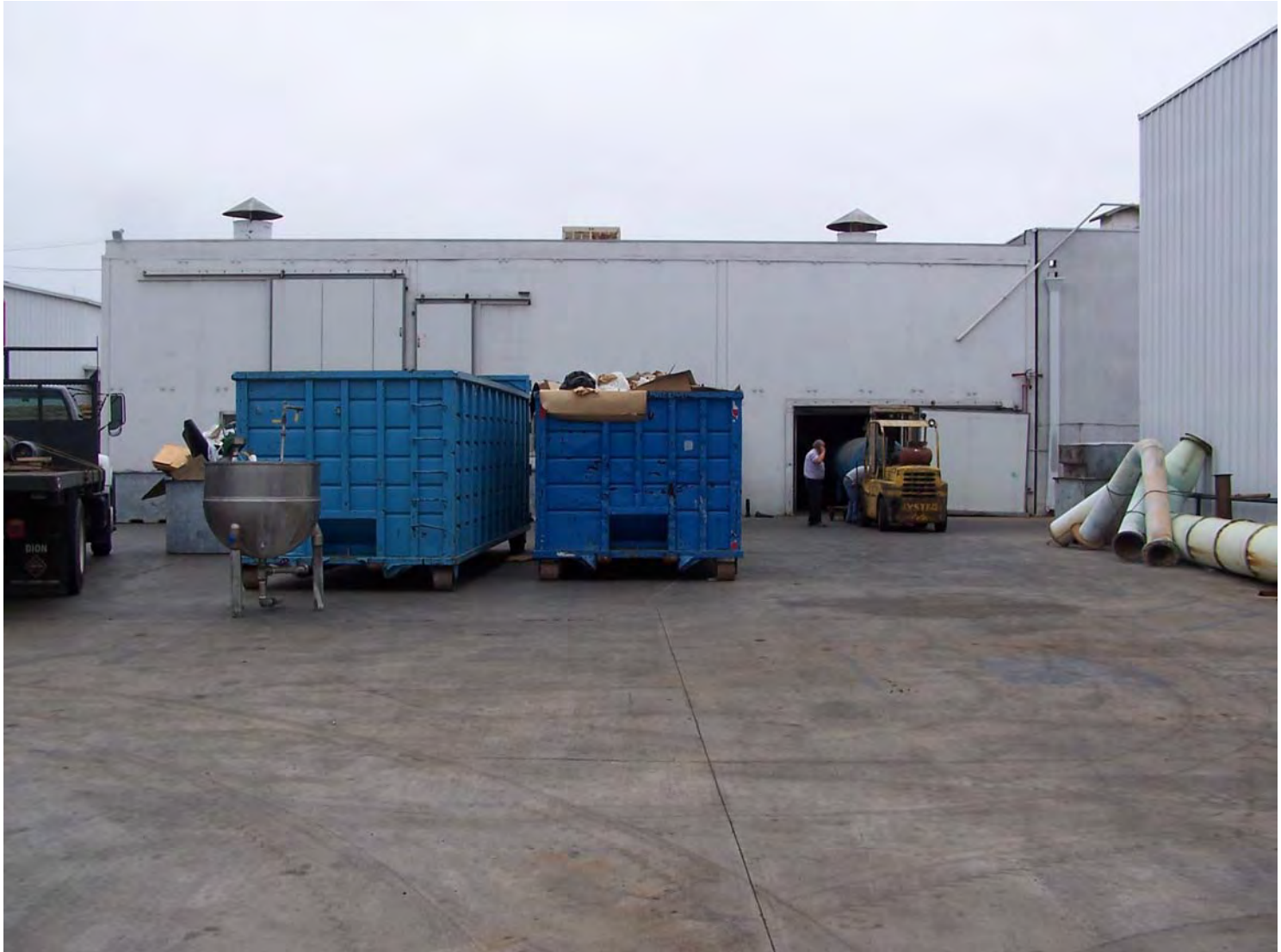
Photograph 1. California Marine Buildings, facing south. 05.02.2006.
