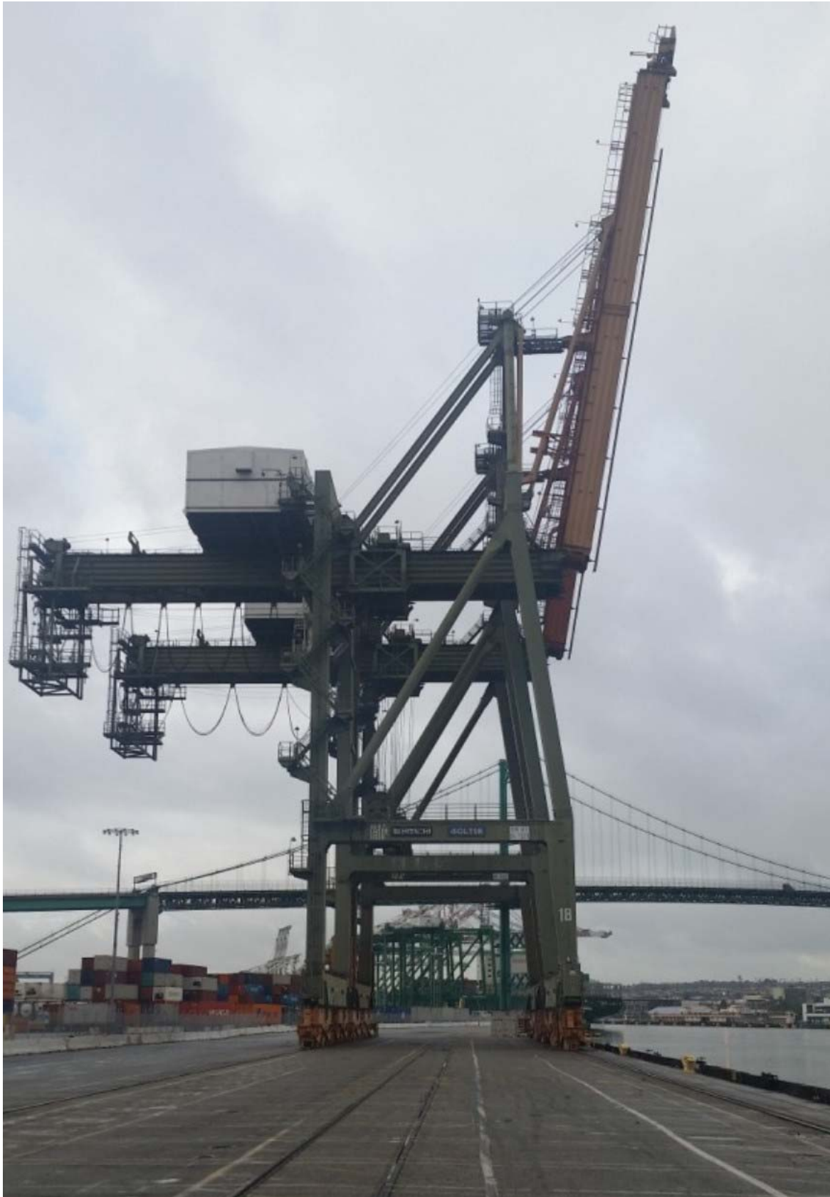
Ship to Shore Cranes 209-18 and 209-19
