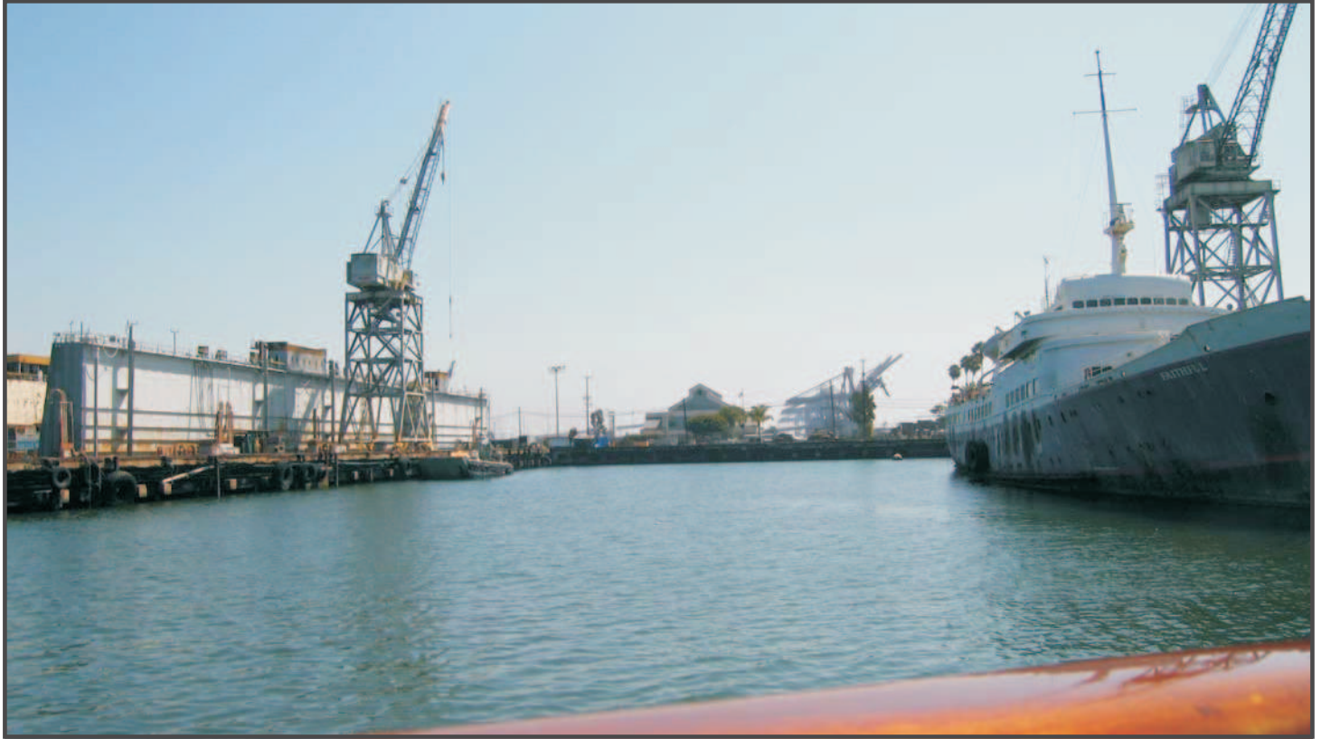
Figure 3.1-1 Near Distance View of Berths 243-245 Slip Fill Site
