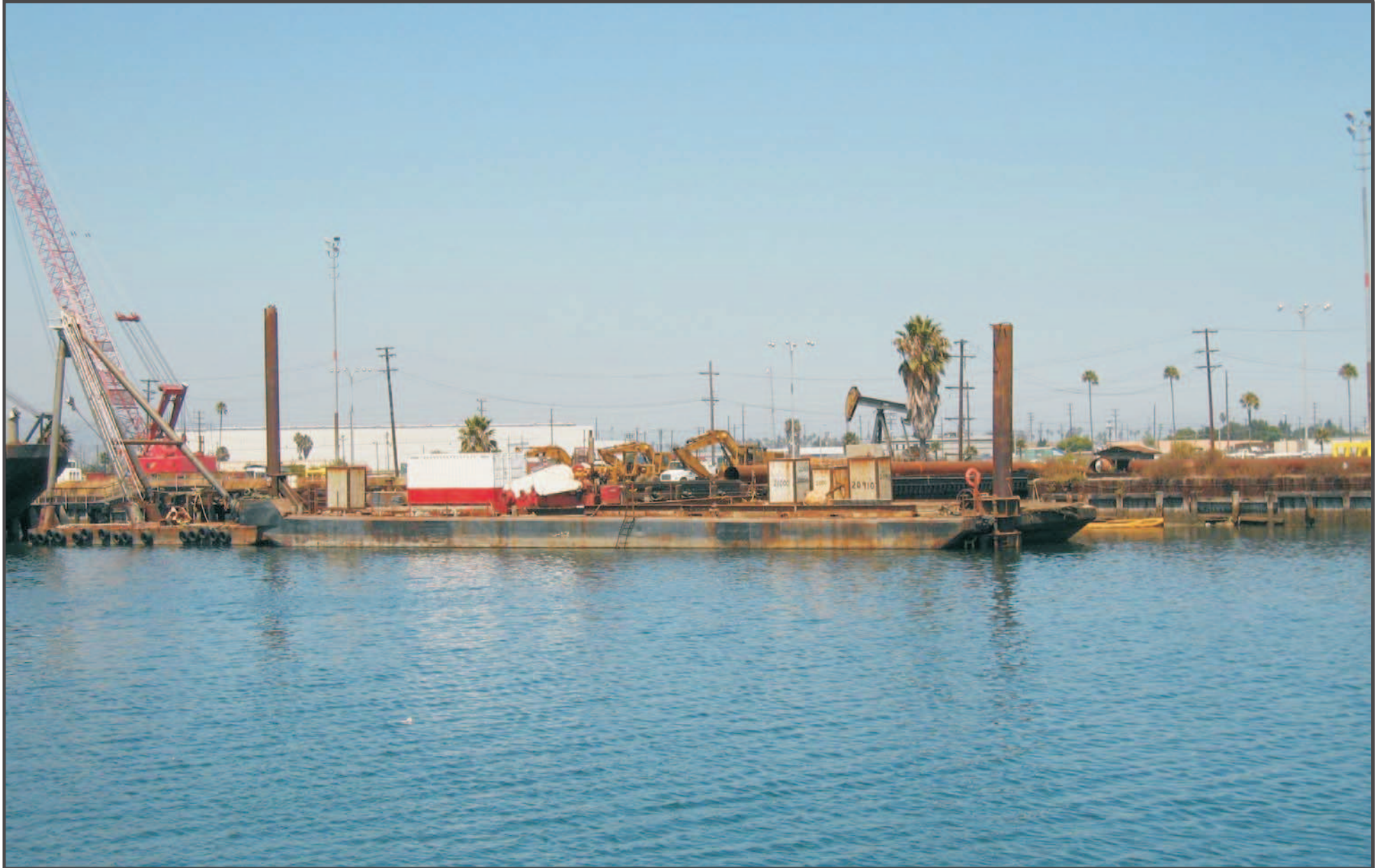
Figure 3.1-3 Northwest Slip Middle Distance View
