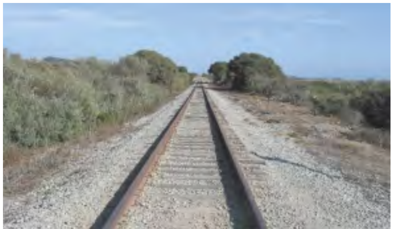
Railroad corridor, Santa Cruz County
