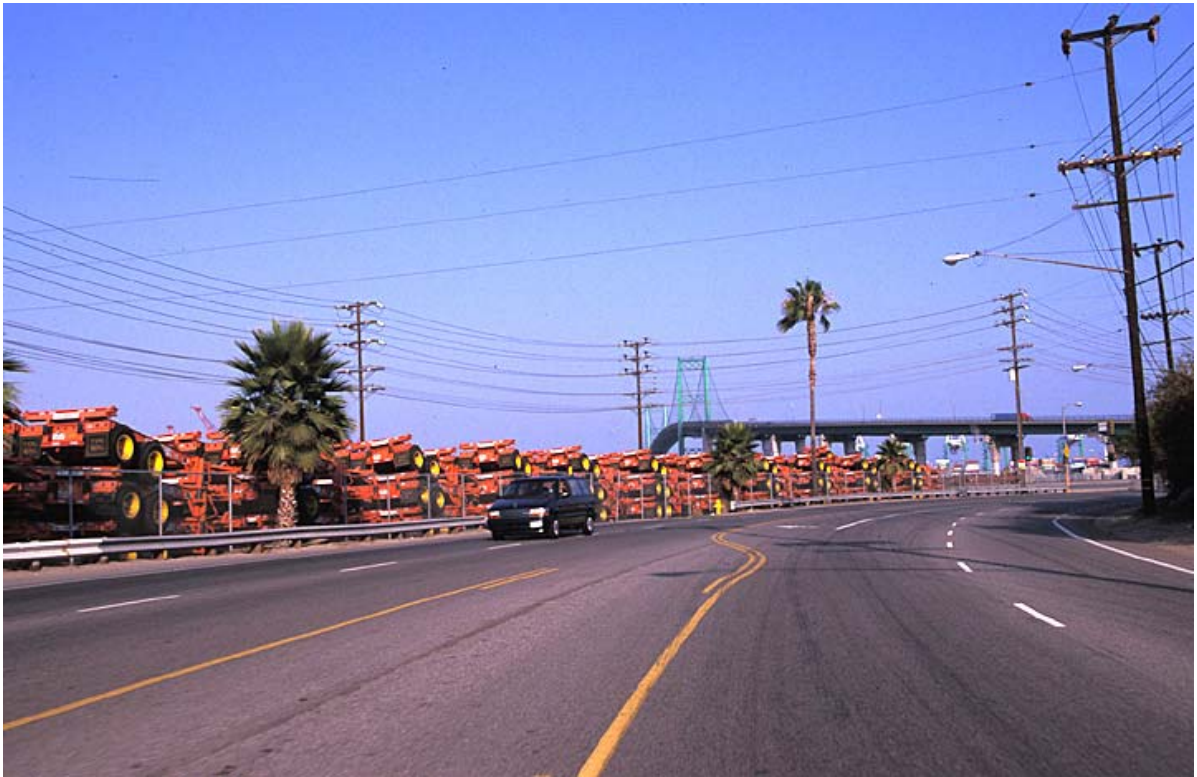
Photograph 11 - View of the Project site and the Vincent Thomas Bridge from the southbound lanes of Front Street.
