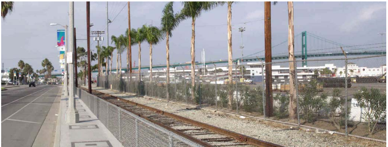
Photograph 12 - View from the northbound lanes of Harbor Boulevard in the area south of the World Cruise Center. The Project site lies on the other side of the Vincent Thomas Bridge.
