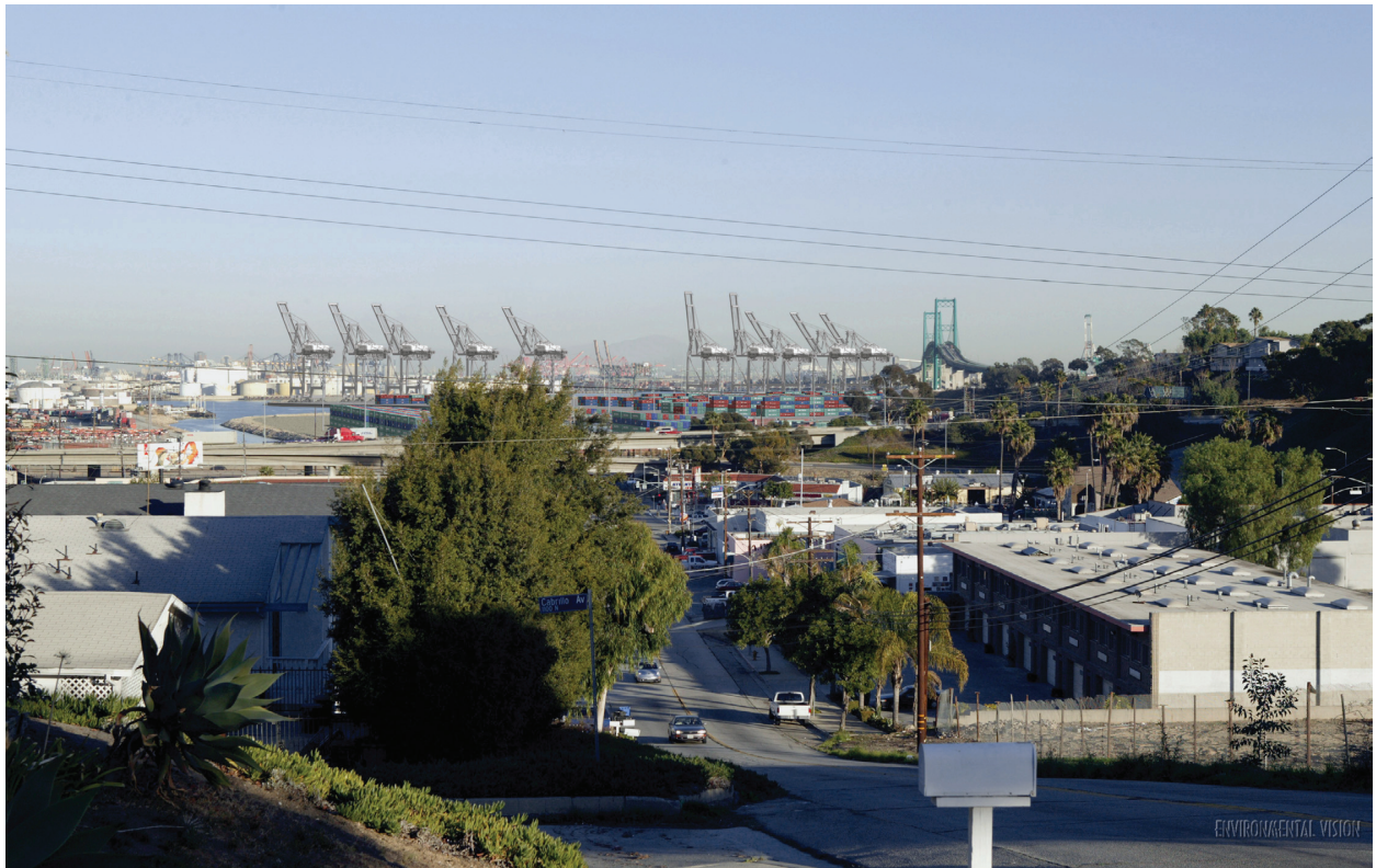
b. Visual simulation of proposed Project with gray cranes seen from Channel Street, as proposed under Mitigation Measure AES-2
