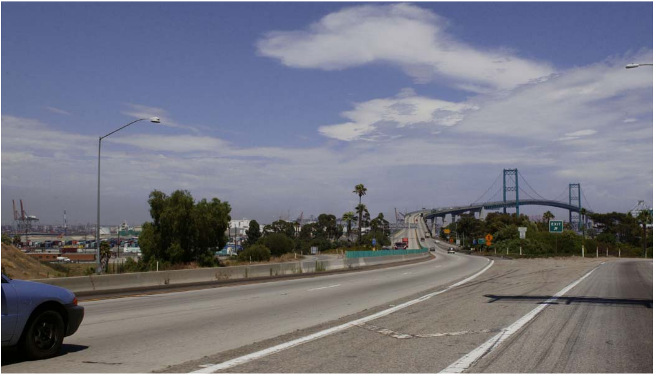
a. Baseline conditions view from SR 47 looking east
