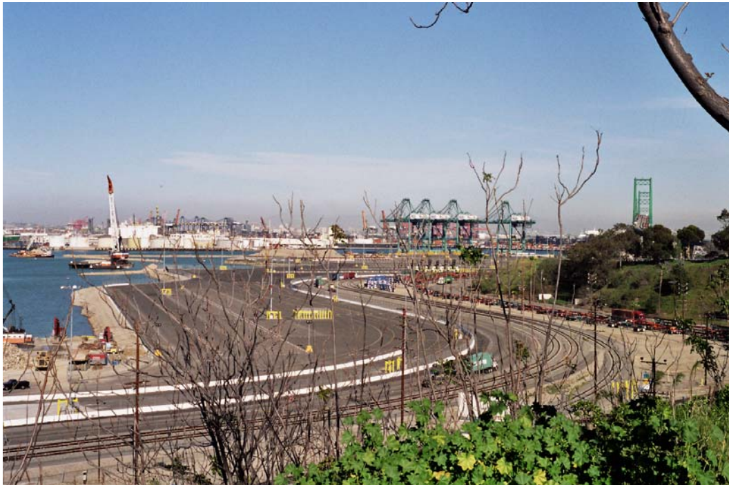
Photograph 16 - View from Shields Drive toward the Vincent Thomas Bridge and the four post-2001 cranes.
