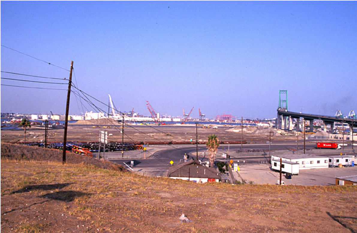
Photograph 3 - View of project site from Knoll Hill
