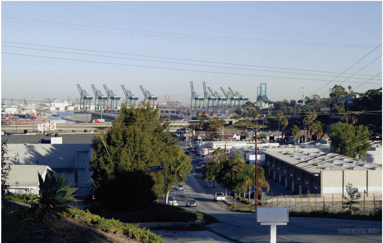
a. Visual simulation of proposed Project with green cranes, as seen from Channel Street
