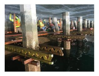
226-236, **Everport Berths Container** Terminal Improvements – Construction continues at this terminal to deepen berths and improve terminal facilities to accommodate larger next-generation vessels. The project involves improvements at Berths 226-229, increasing berth depth from -45 to -53 feet, and improving Berths 230-232 to a -47 feet berth depth. The project also involves constructing an additional 1.5 acres of backland and electrical
